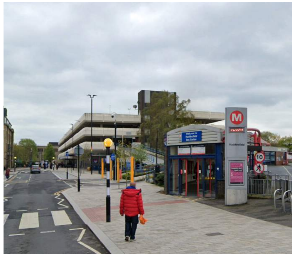
View from the north entrance on Upperhead Row
