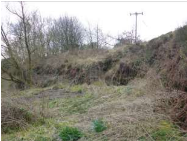
Photo 3: The quarry face is present along the western and southern sides of the quarry and is mostly vegetated.
