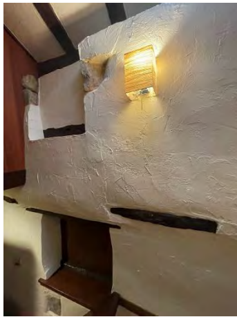
Photo 3: Blocked openings within the southern end of the byre, facing northeast
