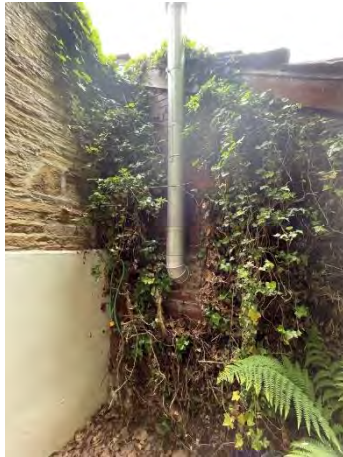
Photo 13: Brickwork to the rear (west) elevation of the garage
