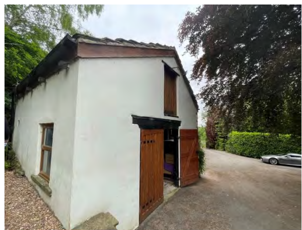
Photo 12: South and east elevations of the garage extension
