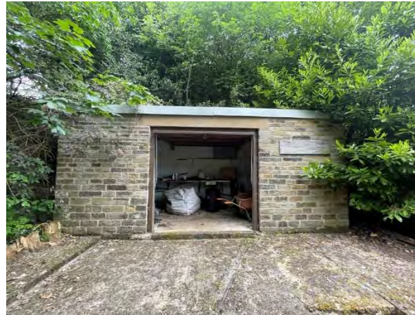
Photo 14: East elevation of the modern outbuilding
