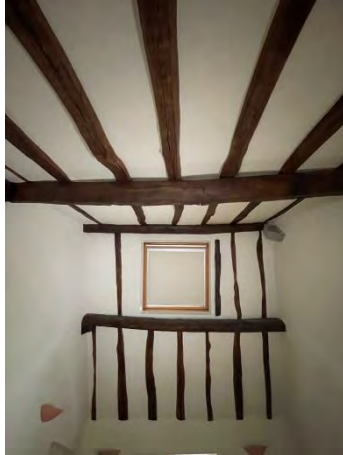
Photo 7: Roof construction within the northern part of the longhouse
