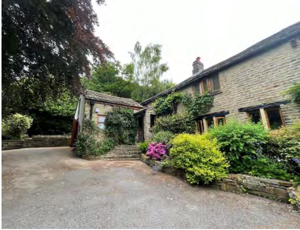
Photo 1: East elevation of the house
