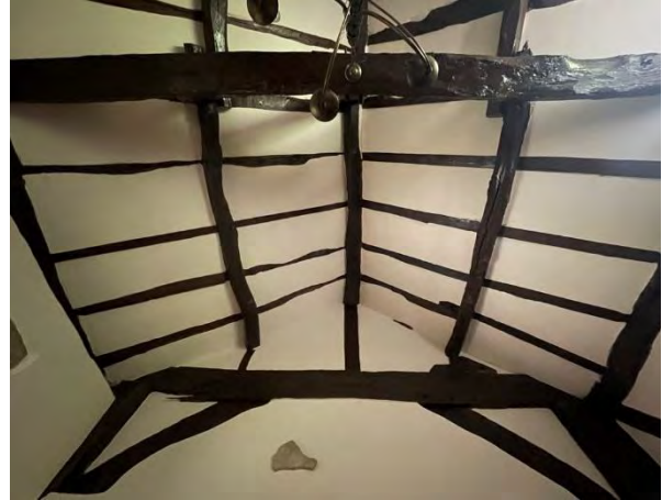
Photo 8: Roof structure above the northern end of the byre
