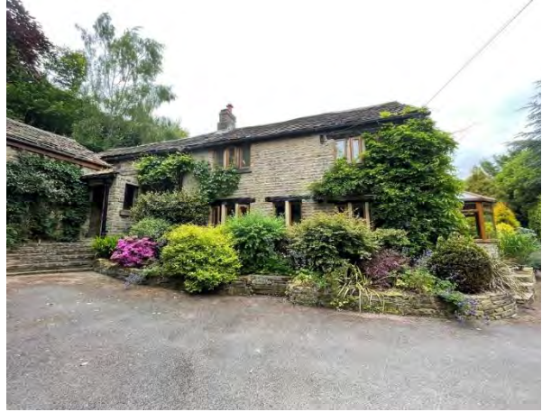
Photo 2: East elevation of the house
