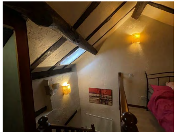
Photo 10: Roof structure above the southern end of the byre, facing southeast
