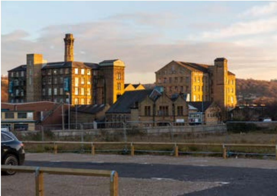
Fig 2.18.1 View east towards Broad Canal
