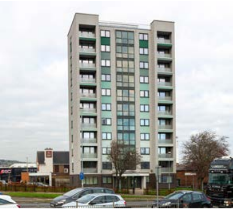
Fig 2.14.2 - Harold Wilson Court, to the North of the site
