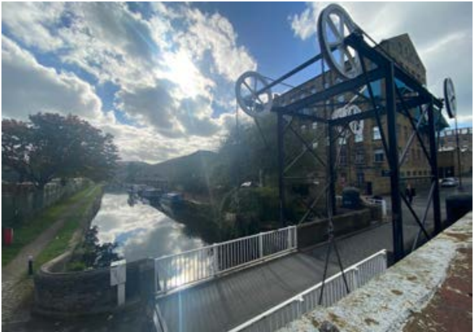
1. Canal bridge over the Broad Canal
