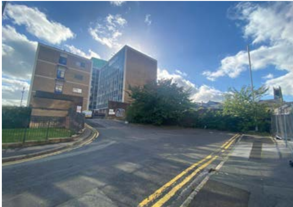
7. View south towards BT openreach building
