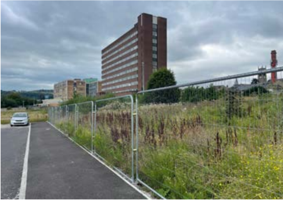
Level changes from Crown House
