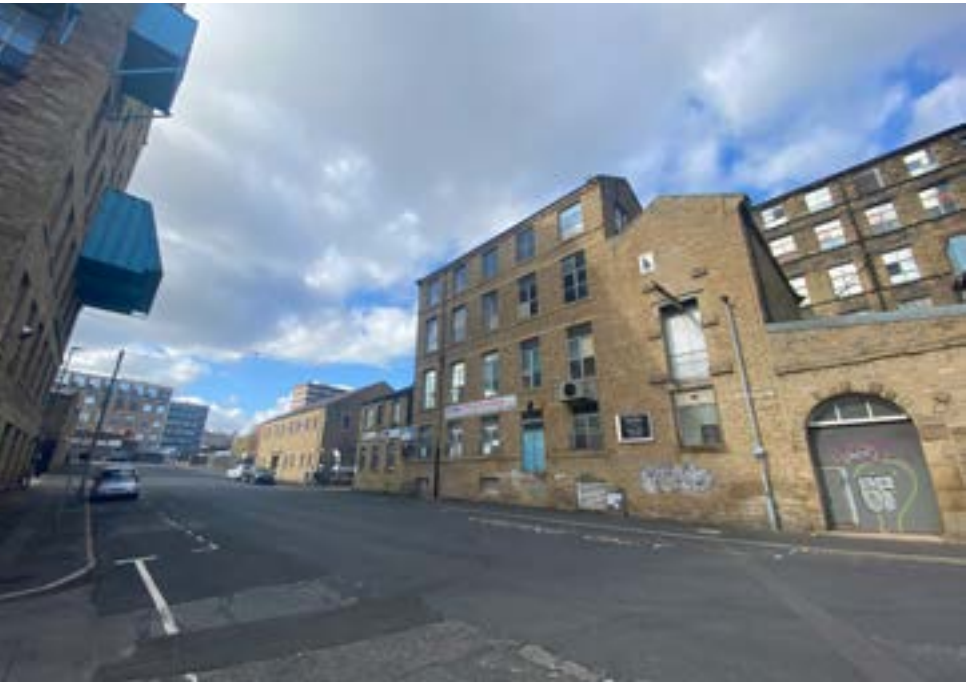
2. View north west down Quay St
