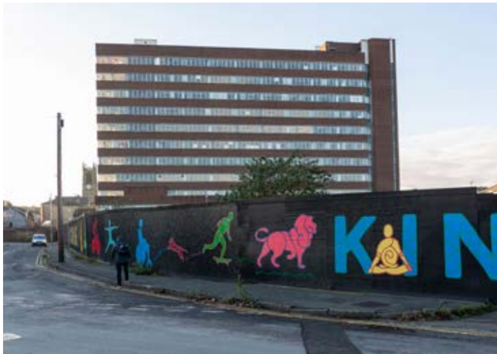
Crown House, to the South of the site
