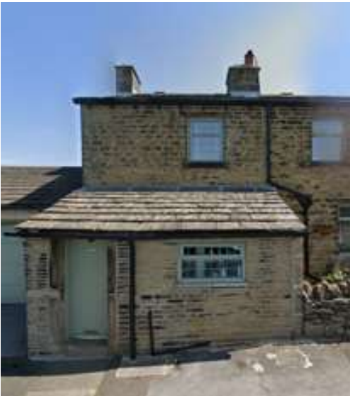
DWELLING AT LINFIT LANE
