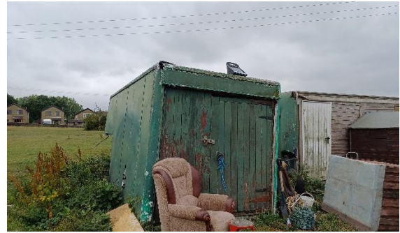
Photograph 14: TN5 – Storage containers (17.07.2025)
