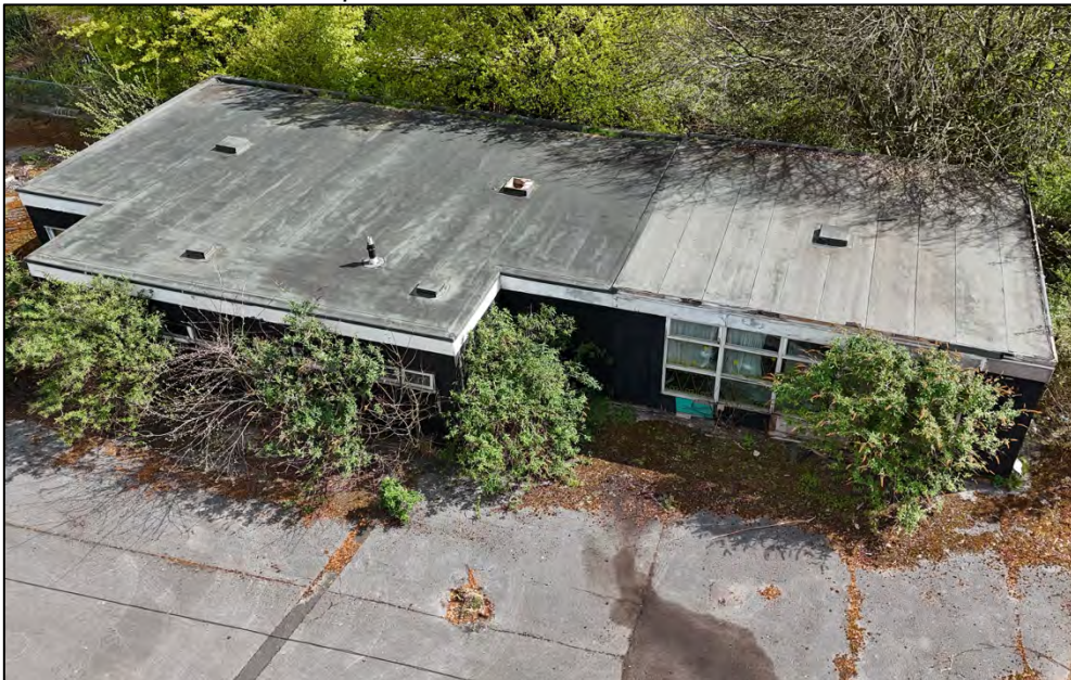
Plate 3: Eastern elevation of B2.
