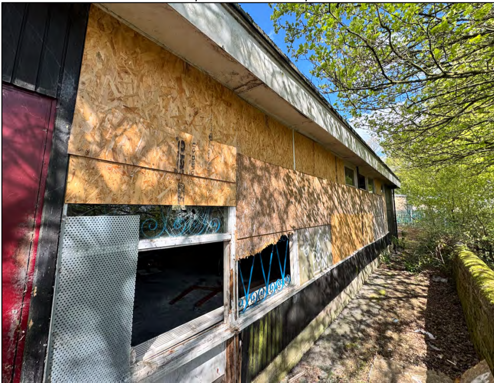
Plate 5: Wooden window boards of eastern elevation of B2.
