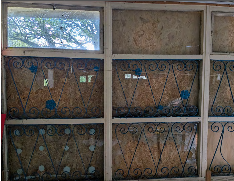
Plate 6: Internal view of wooden window boards on eastern elevation of B2.
