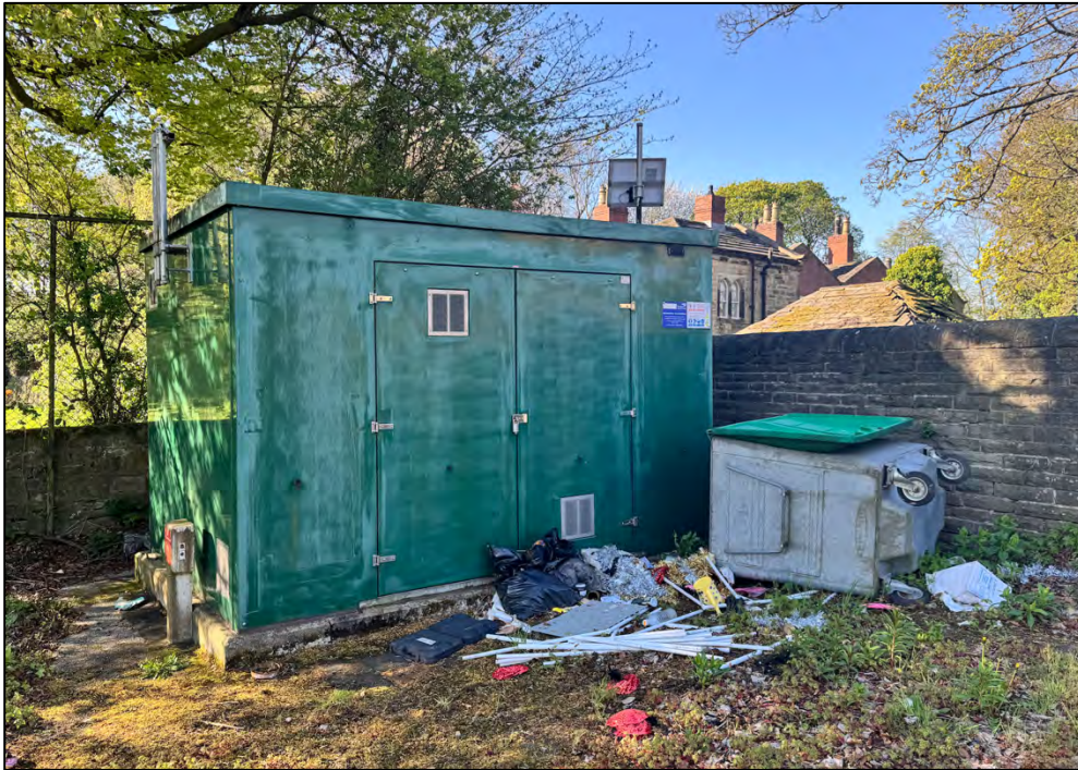
Plate 1: Building 1; Gas services building.
