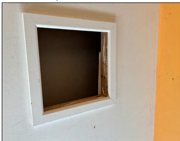
Plate 9: Loft hatch in western room of B2.
