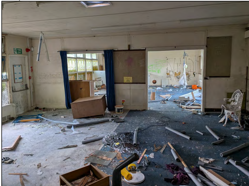
Plate 8: Inside of B2.
