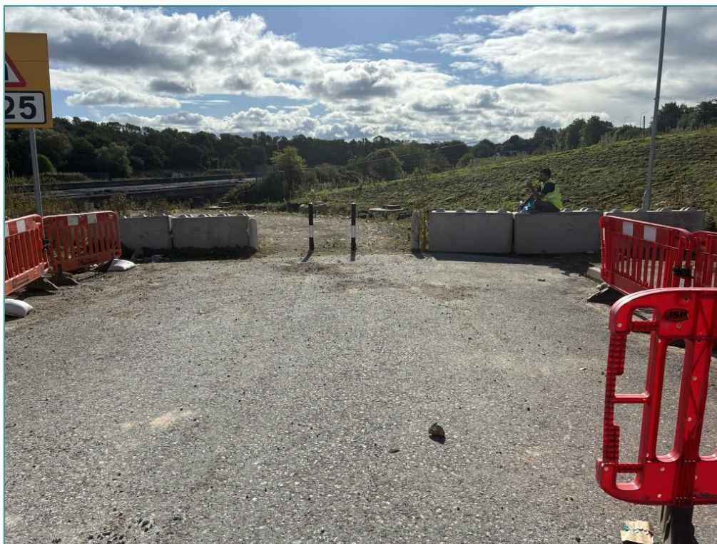
Photograph 1: View Looking South at the Access Road onto Site.
