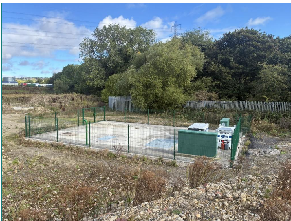
Photograph 9: View Looking at the Adjacent Water Pumping Station.
