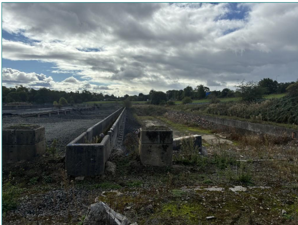
Photograph 5: View Looking South at an Empty Filter Bed.
