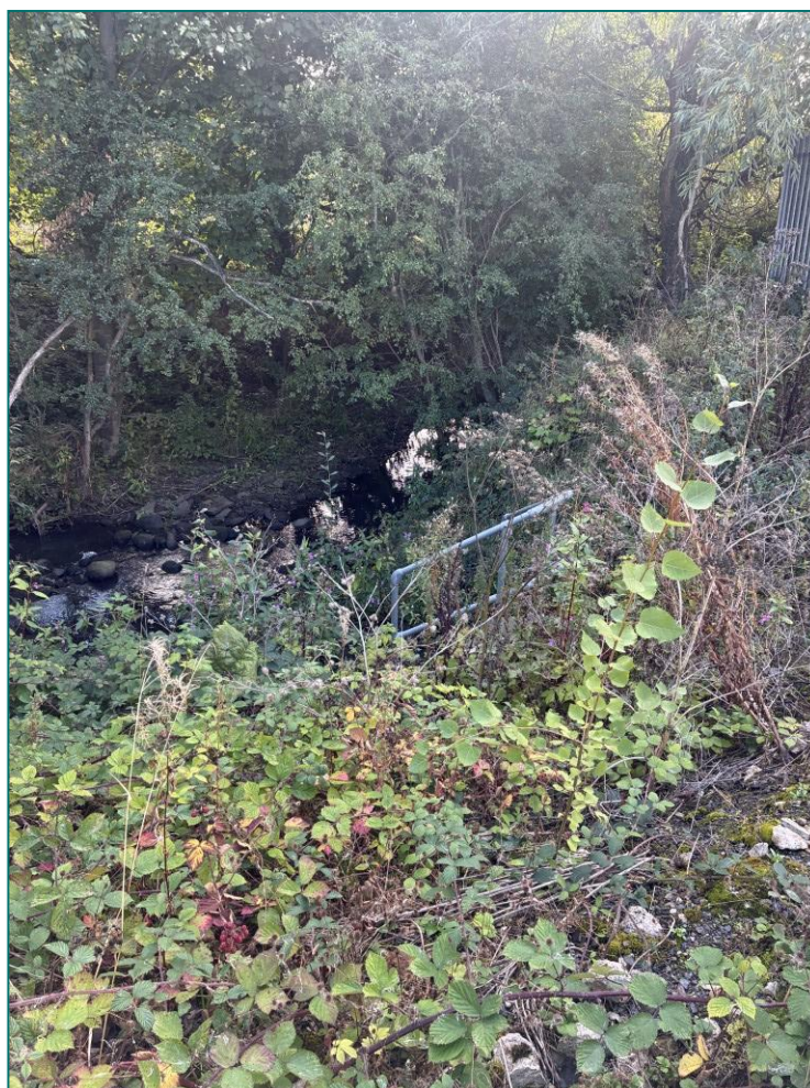
Photograph 10: View Looking at an Outfall into the Hunsworth Beck.
