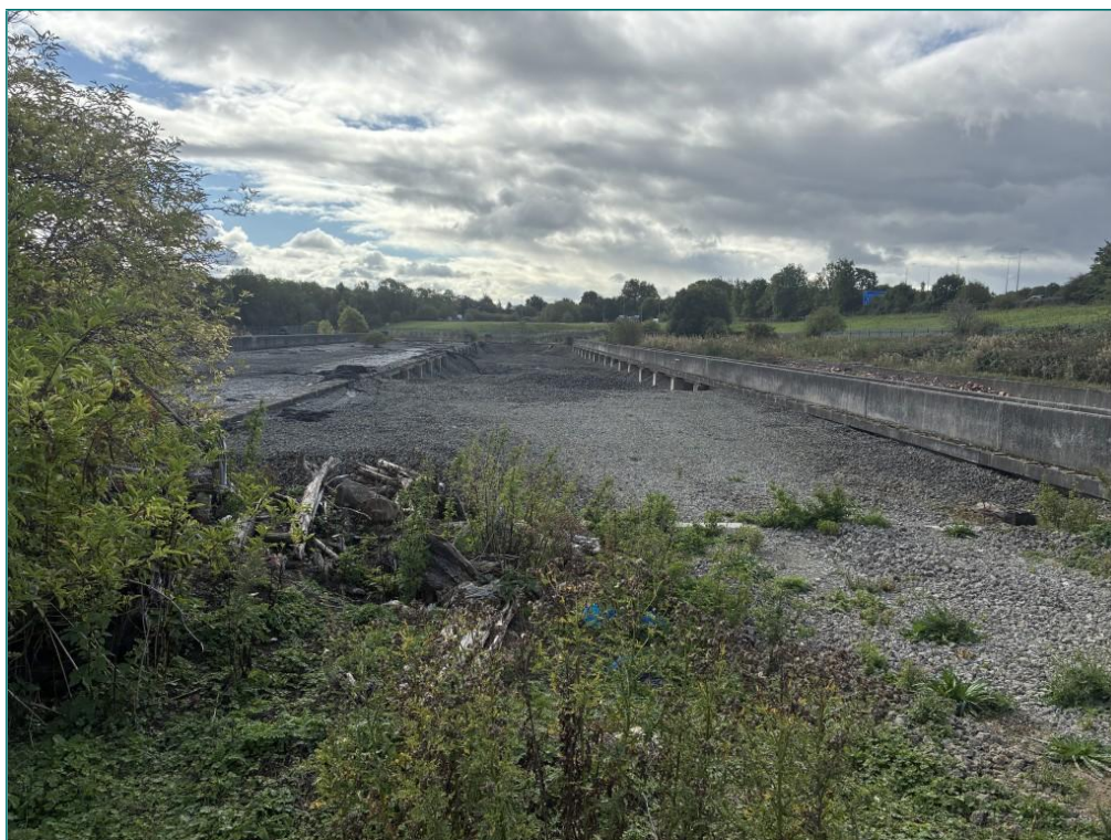
Photograph 4: View Looking South at a Partially Empty Filter Bed.
