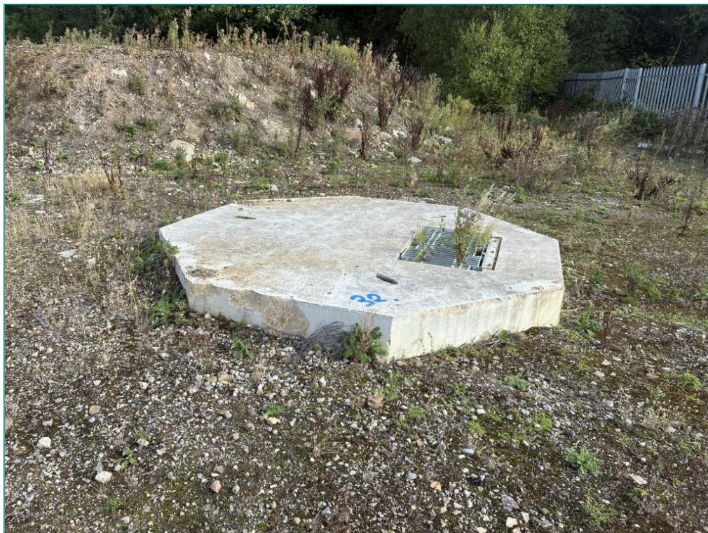
Photograph 12: View Looking at manhole associated with the Pumping Station.
