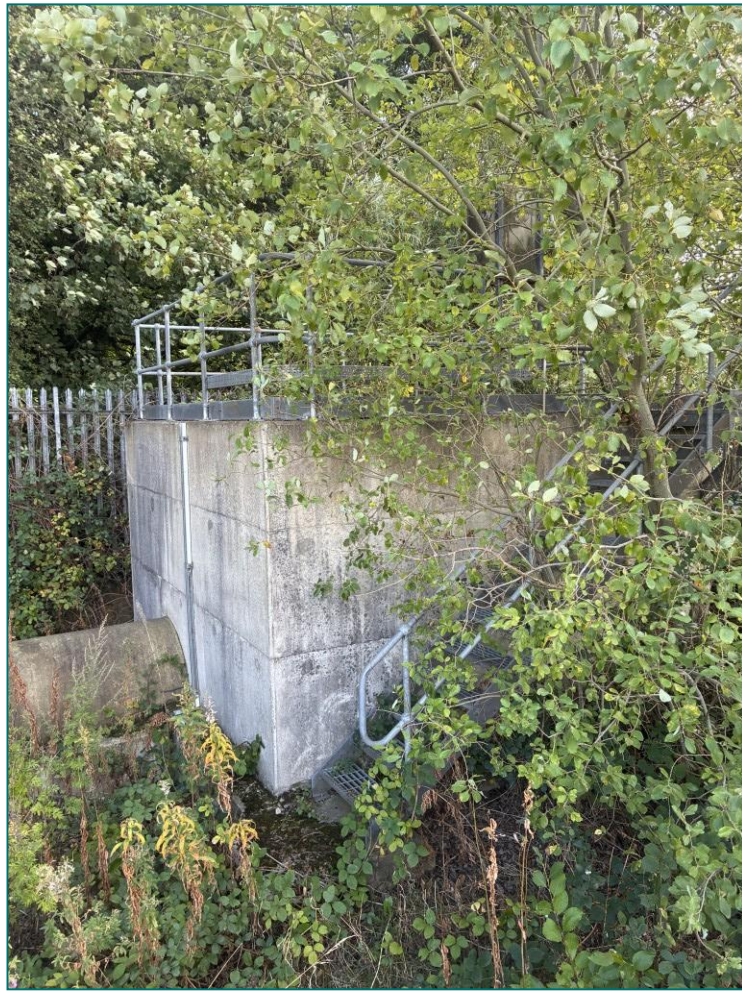
Photograph 11: View Looking at Concrete Utility Structure.
