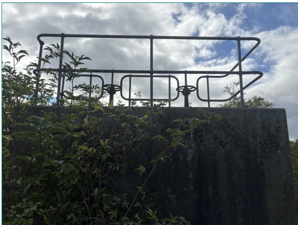
Photograph 6: View Looking at infrastructure associated with the Former Above Ground Storage Tanks.
