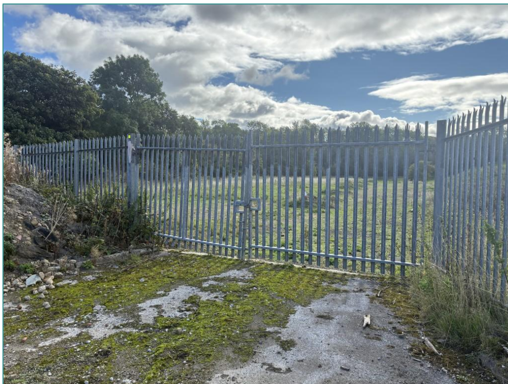
Photograph 7: View Looking at the Palisade fencing and Locked Gate, trending east to west, in the centre of the site.
