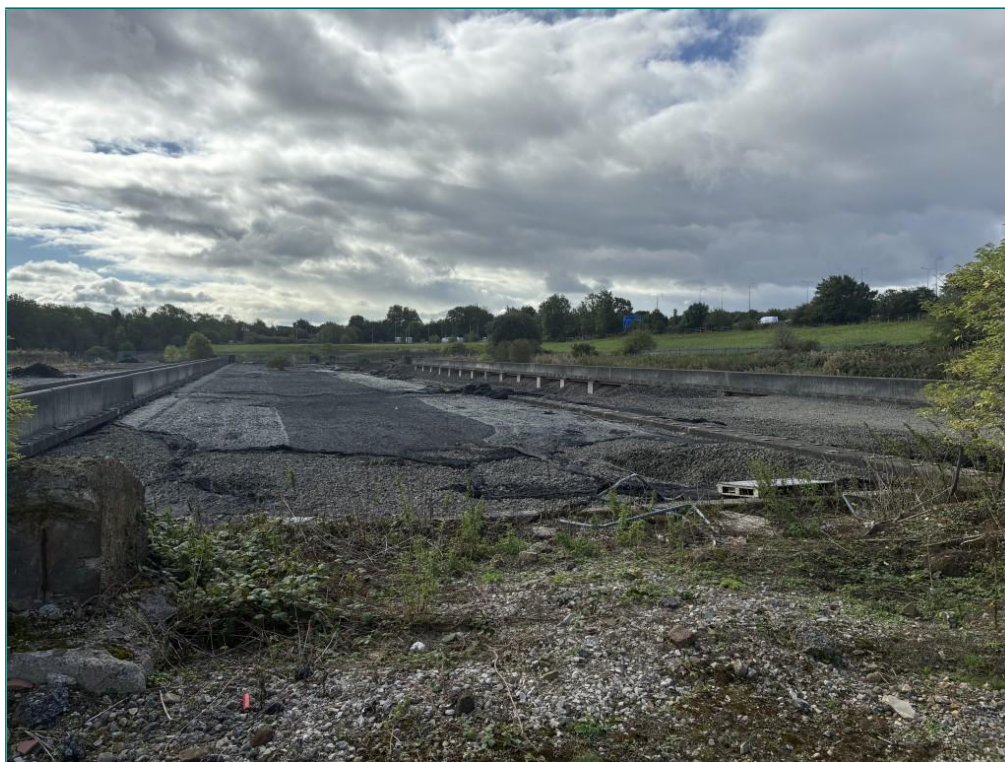
Photograph 3: View Looking South at Second Full Filter Bed.
