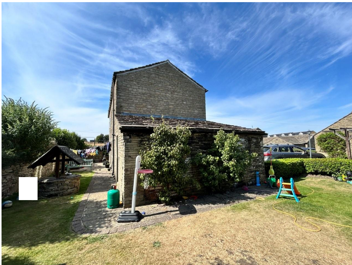
Gable (southeast) elevation
