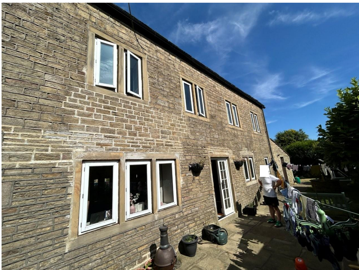
Rear (southwest) elevation
