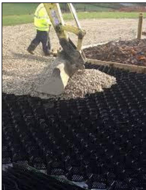
Figure 4.4: Cellweb® geo-cellular confinement sheets being installed.
