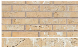
Example of facing Brickwork.
