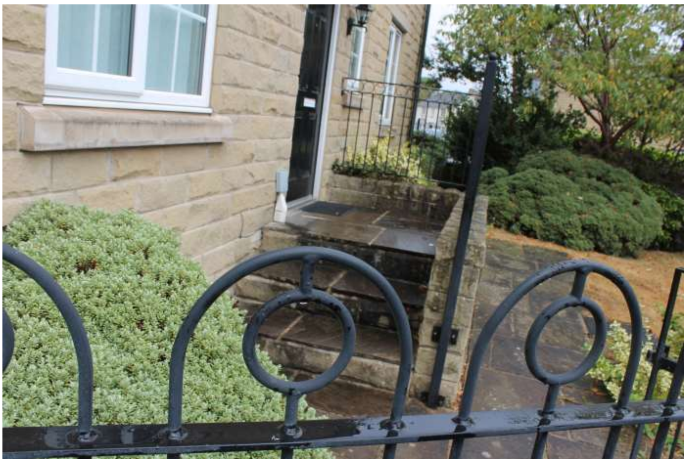
Existing front access steps
