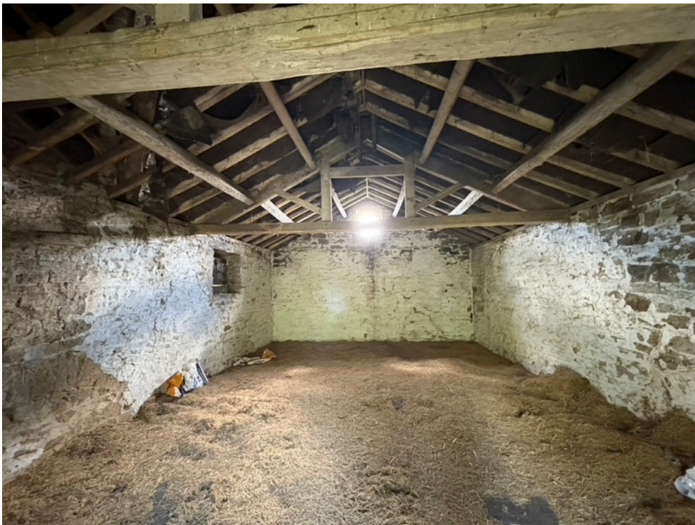
Internal photo at first floor towards south east
