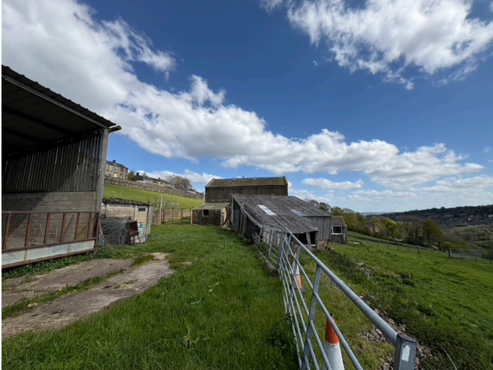
View of barn with existing outbuildings
