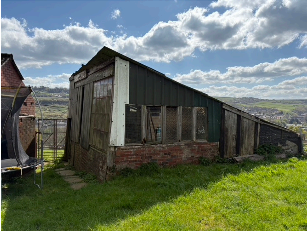
Outbuilding immediately in front of barn (to be demolished)
