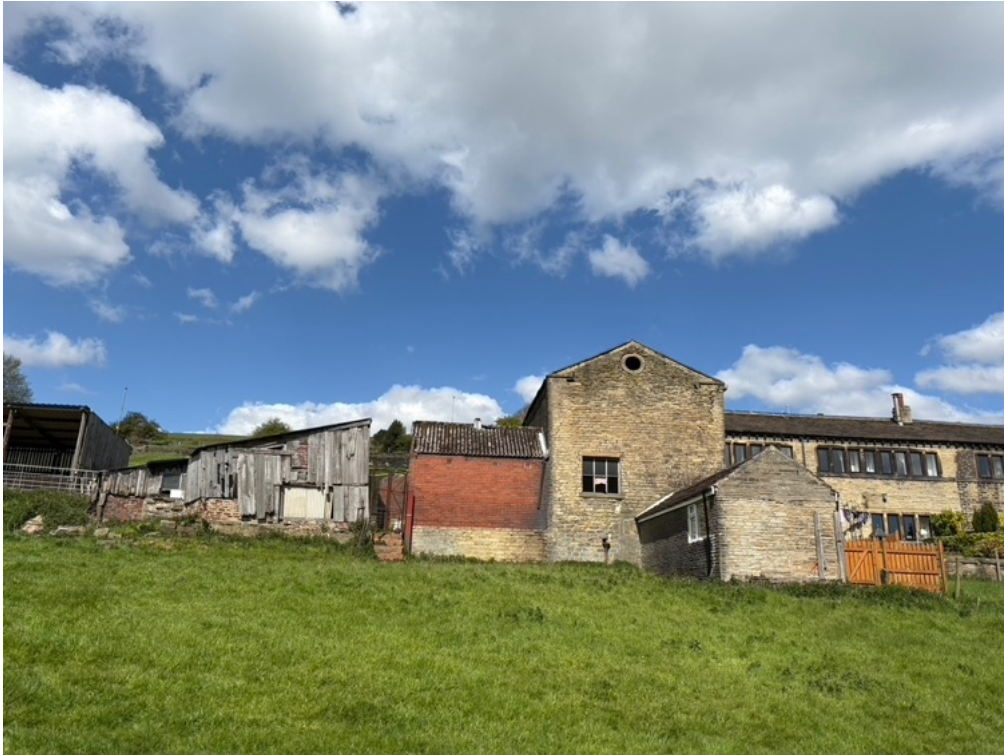
South east elevation / external building
