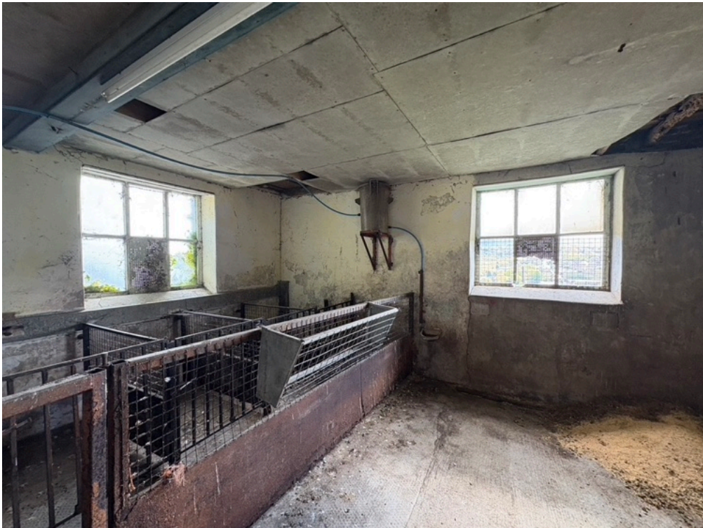
Internal photo at ground floor towards south east
