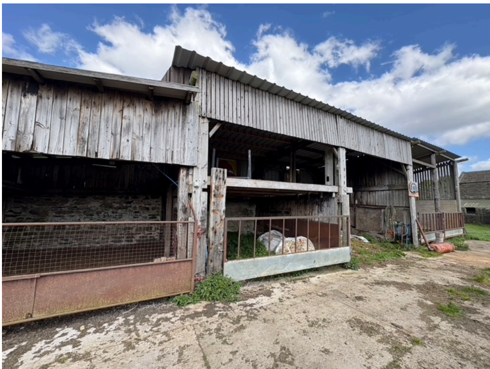
Agricultural structures retained (other than end bays noted above).
