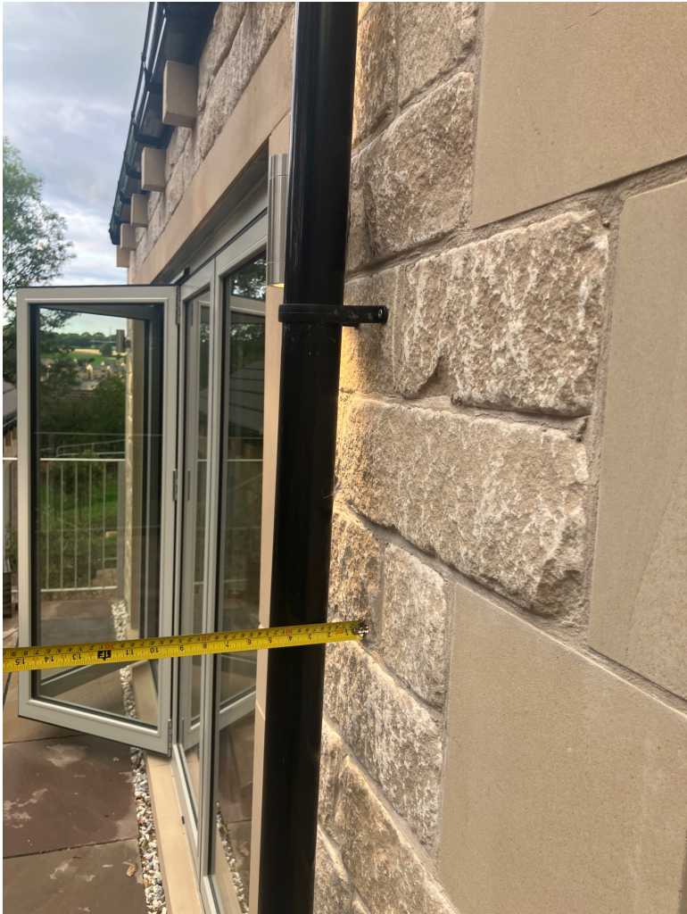
Photo 2 – Existing rainwater downpipe and rear wall.
