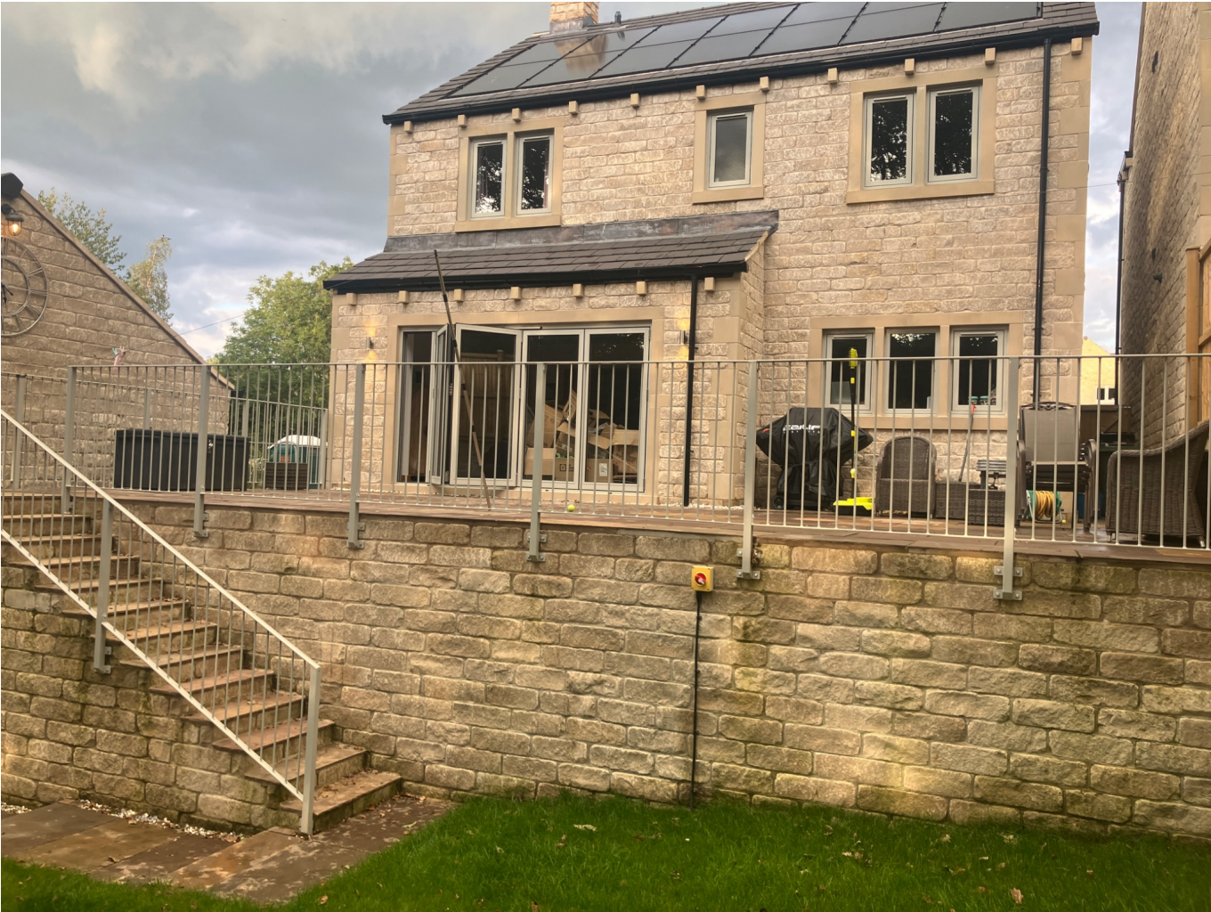
Photo 1 – Existing rear elevation, raised paved terrace and lower garden.
