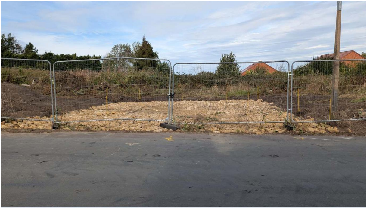
Photographic record of construction works undertaken to the site access, representing a material start and lawful implementation of Planning Permission 2026/70/90373/E
