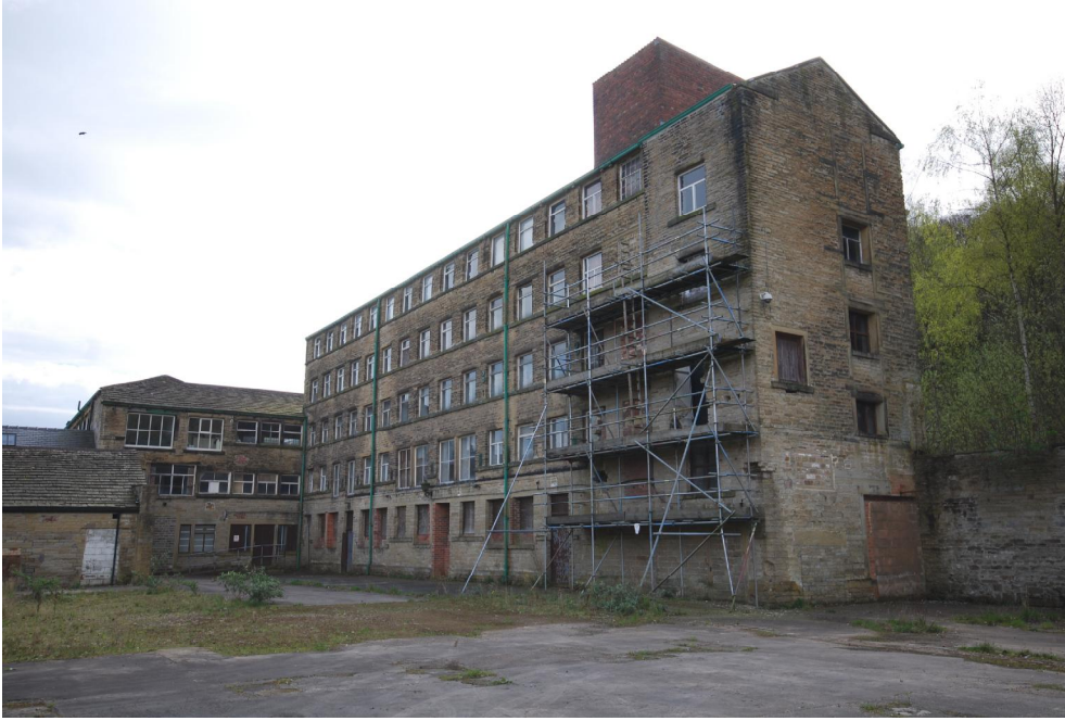
4.10. The North side of the 1830 Loomshop (8) Building 29, linking to the earlier hand spinning and weaving shop in the background.
