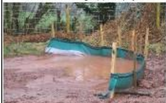
Hy-Tex Terrastop silt fence in use on National Grid's Felindre to Brecon gas pipeline project
