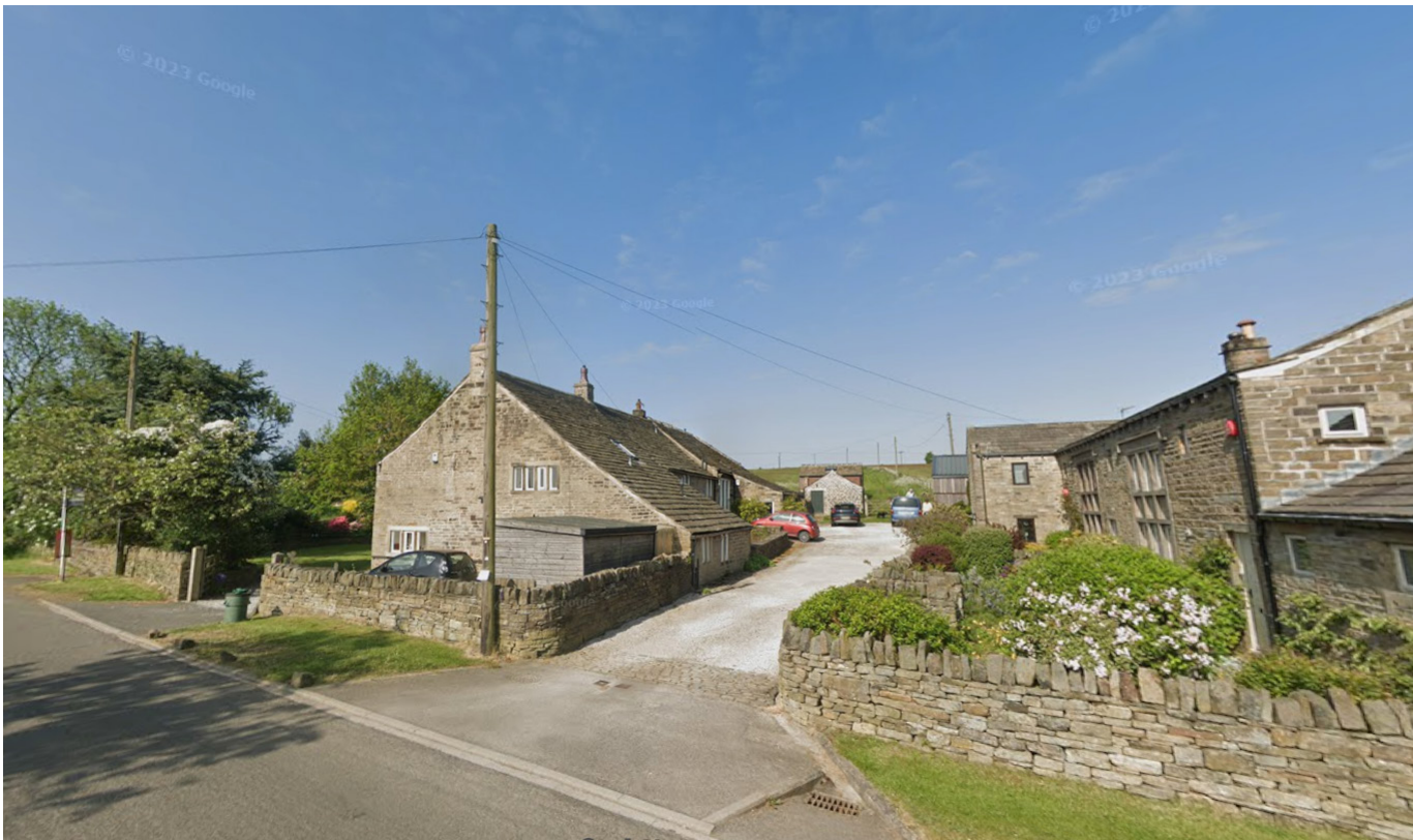
View looking southwest into the site from Marsh Hall Lane.
