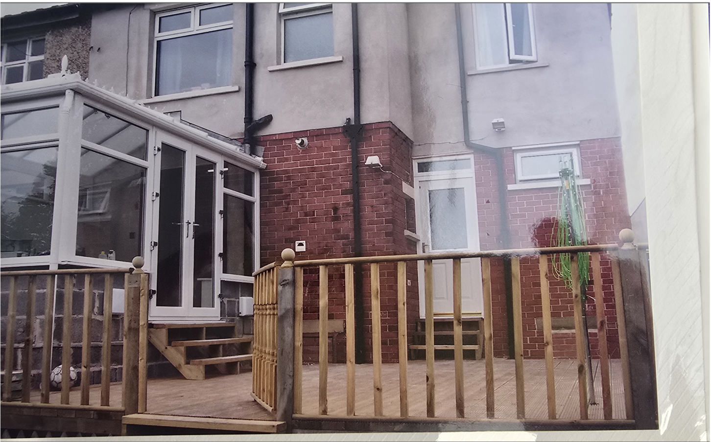
Decking built on top of patio area 2011
