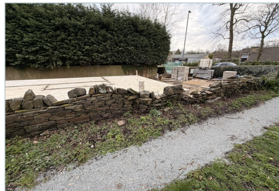
Photo 6 - 26 March 2026. Surviving wall lengths are reduced and disordered after progressive site works.
