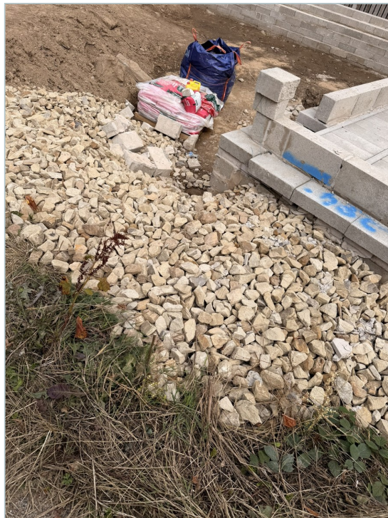
Photo 2 - close view. Floor units/substructure and corner blockwork, with the adjoining driveway level visible.
