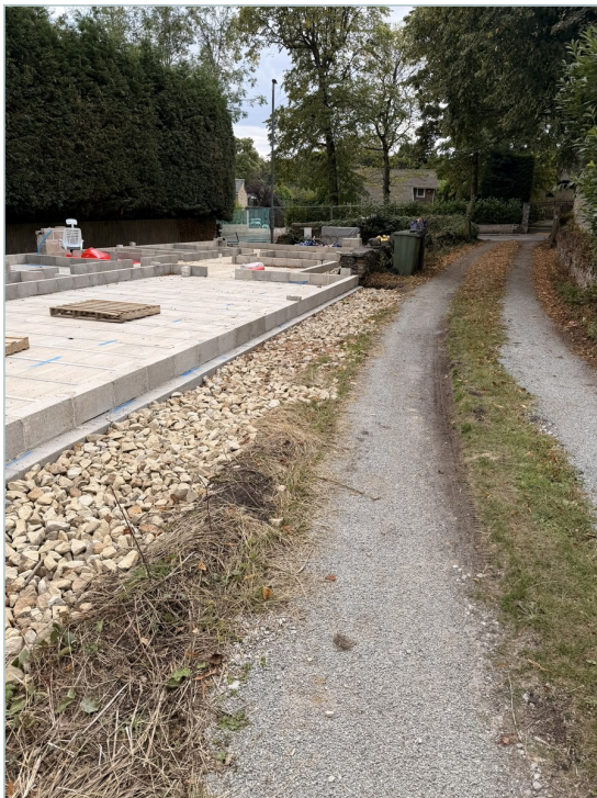
Photo 1 - wider view. Completed suspended floor deck/substructure and low perimeter blockwork beside the access drive.
