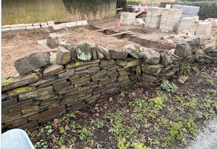
Photo 3. Existing dry-stone wall beside the development and access.
