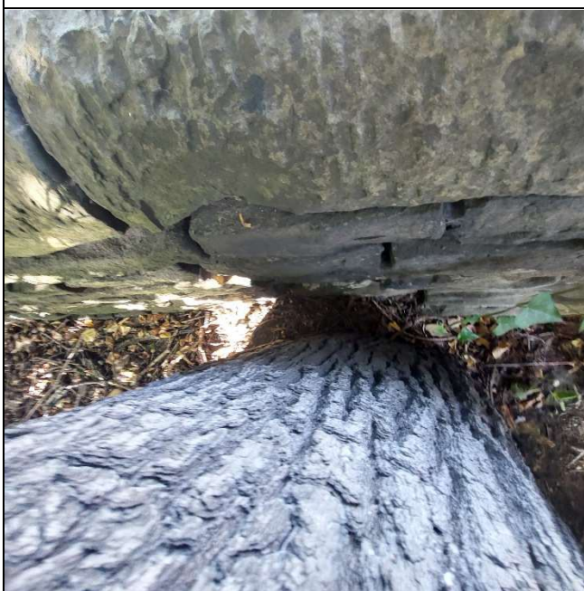
Photo 7 and 8: T5 Pedunculate Oak. The west side of the tree's buttress is against the boundary wall and when viewed outside the wall was seen to bowing slightly.
