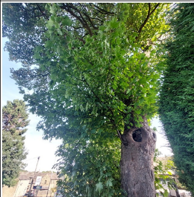
Photo 4: T4 Sycamore. Two branch wounds with cavities forming looked acceptable at present.
