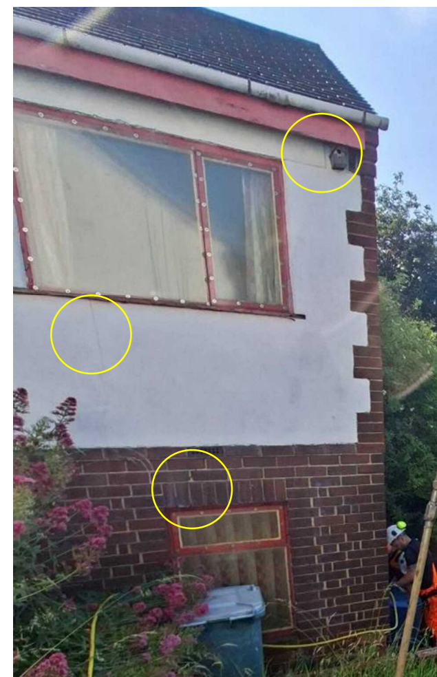
Photograph 2: General presentation of existing structure with minor cracking circled in yellow + drilling RO102
