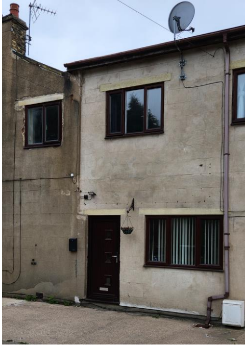
Figure 4 North Facing Elevation View
