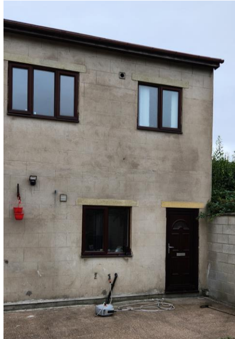
Figure 5- North Facing Elevation View 2
