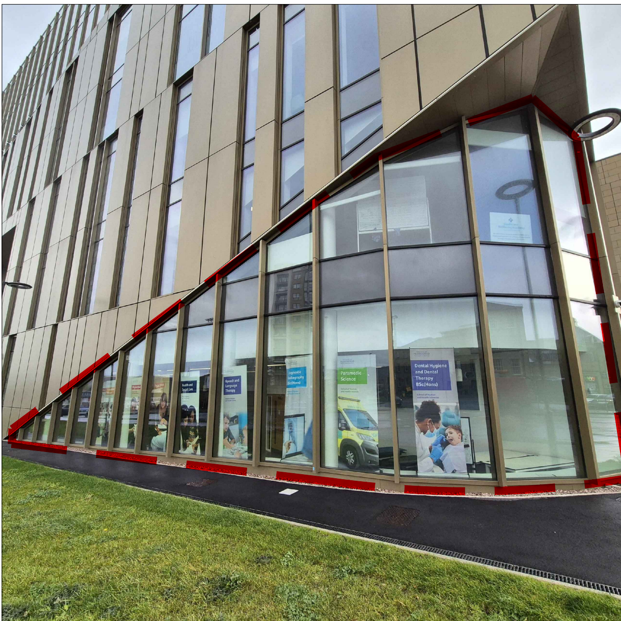
pic 1, VIEW ON EXISTING GLAZING / SOUTHGATE / SIDE
