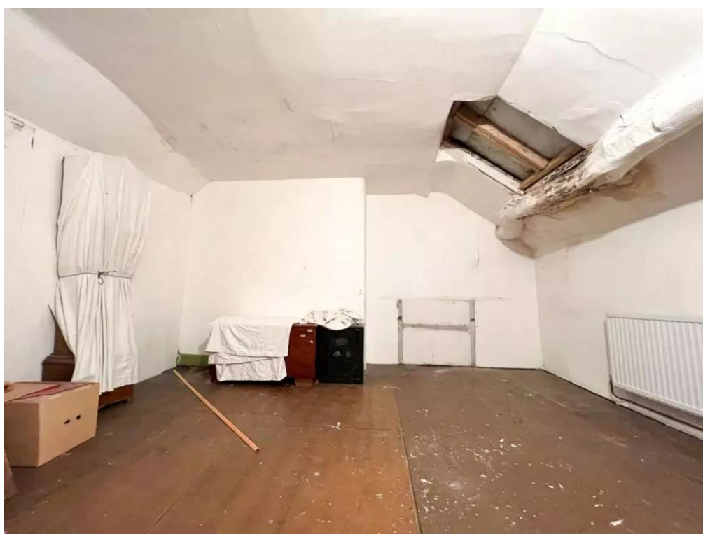
Internal photo showing the current conditions of the existing roof
