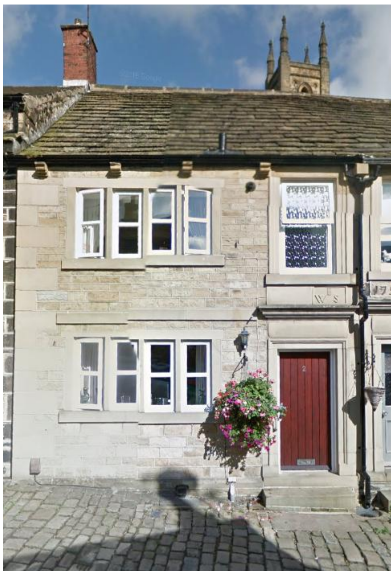
2 Exchange – photograph from 2016 showing timber door and windows – the photo on page 1 of this statement from approx. 2024 shows uPVC windows and door, reflecting that there has been a change
