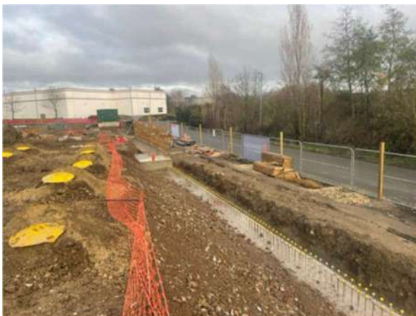
Retaining wall progress
