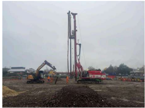
Soil Engineering SM11 rig in progress
