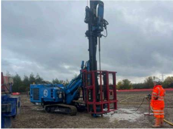
Soil Engineering SM11 rig in progress
