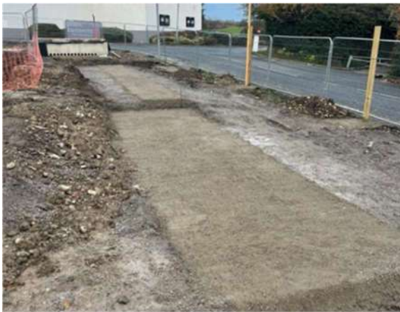
Ground slab for construction of the retaining wall at the south of the site
