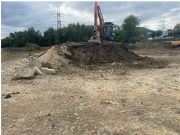
Organic material stockpiled on site
