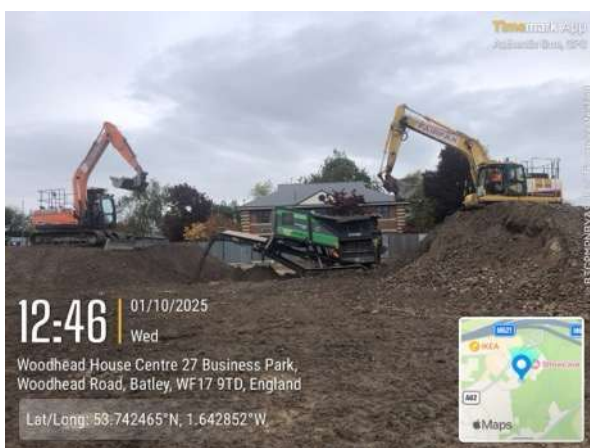
Above left: Crushing material
