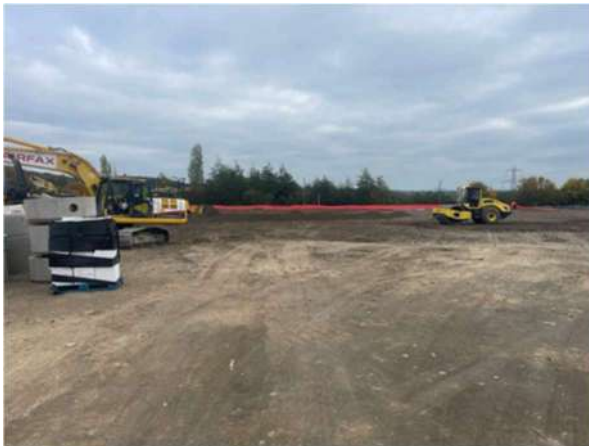
Compaction of fill material
