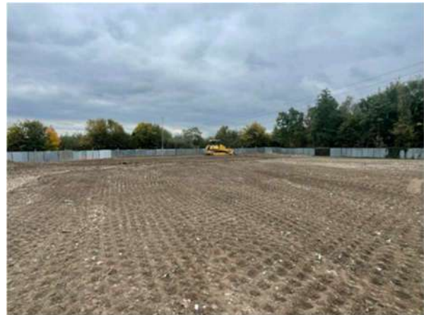
Bottom Right: Levelled site rolled and compacted.
