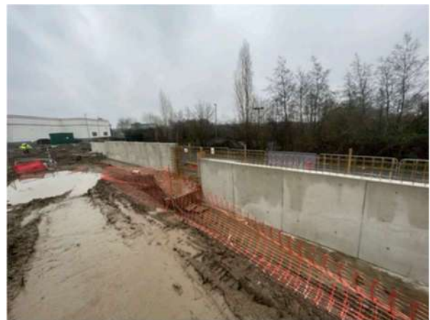
Retaining wall progress
