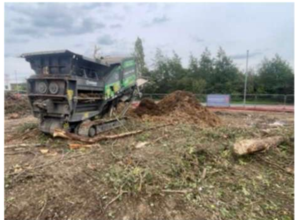
Crushing/grinding excavated organic material
