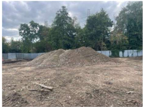
Graded crushed concrete
