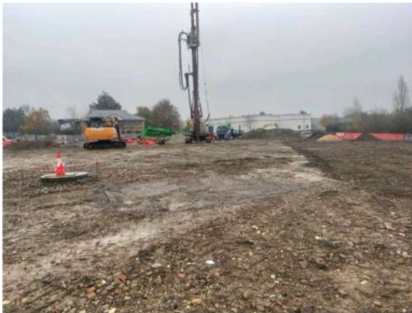
Soil Engineering SM11 rig in progress
