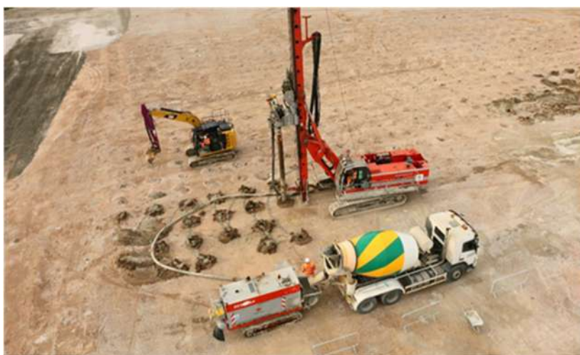
Figure 4 - CMC setup on site
