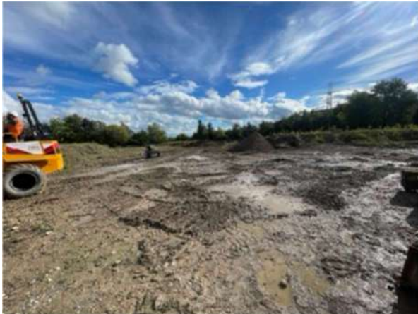
View across the site during site setup and topography survey
