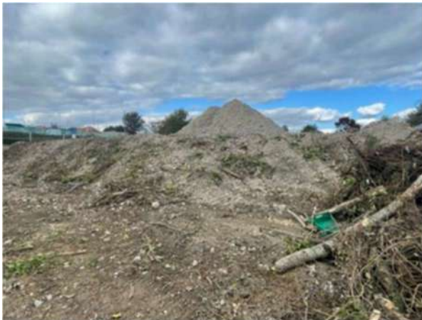
Stockpile of existing crushed concrete to be graded
