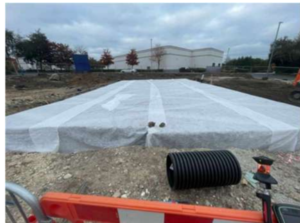
Attenuation tank installation prior to backfill and surround
