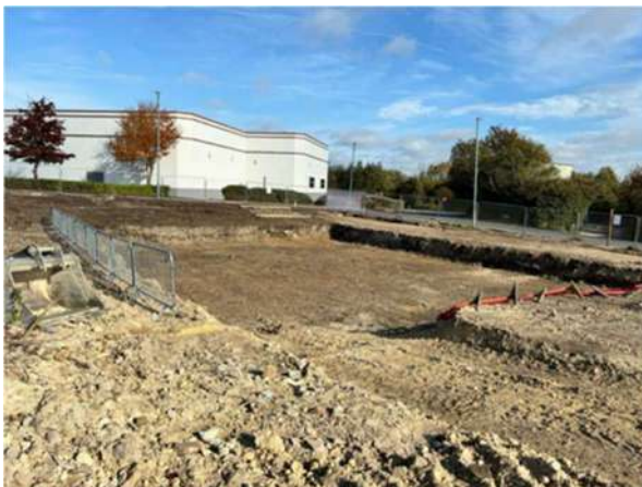
Excavation of attenuation tank in progress
