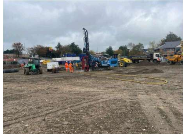
Soil Engineering SM11 rig in progress
