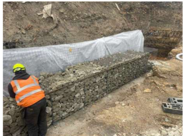
Progress of gabion wall in the western corner
