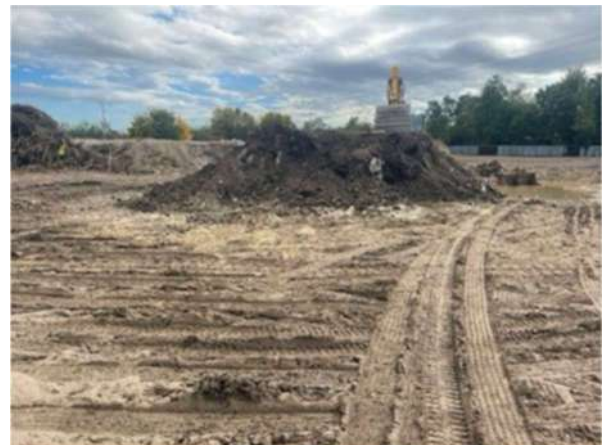
Stockpile of remaining organic material to be removed from site
