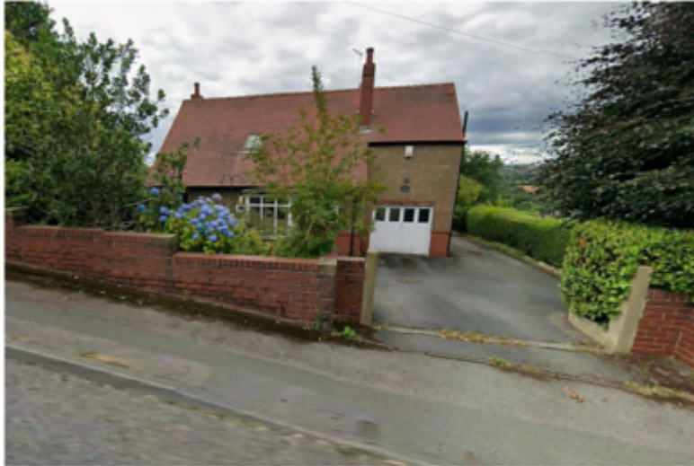
5 Far Bank – Existing dwelling
