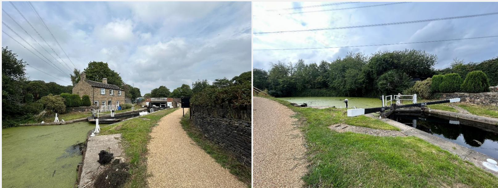
Image 7.1: Grade II Listed Keepers Cottage and Cooper Bridge Lock
