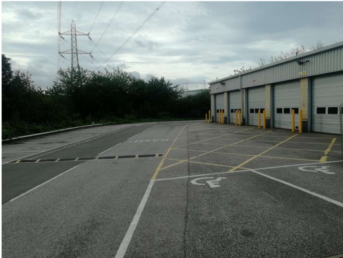
Photograph 5: Area of hardstanding at eastern end of the site, facing south.
