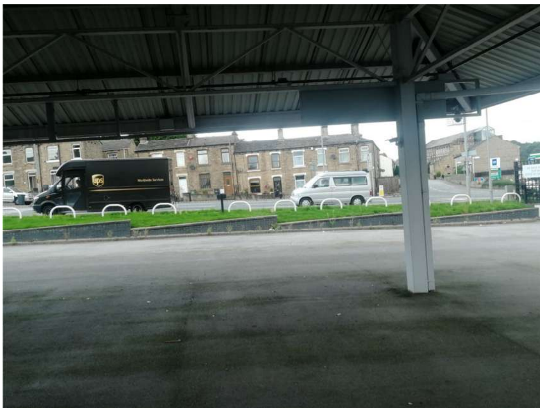
Photograph 20: Open sided canopy at northwestern boundary, facing northwest.
