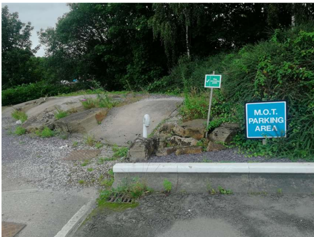
Photograph 4: Area of crushed slate surfacing at northern boundary, facing north.
