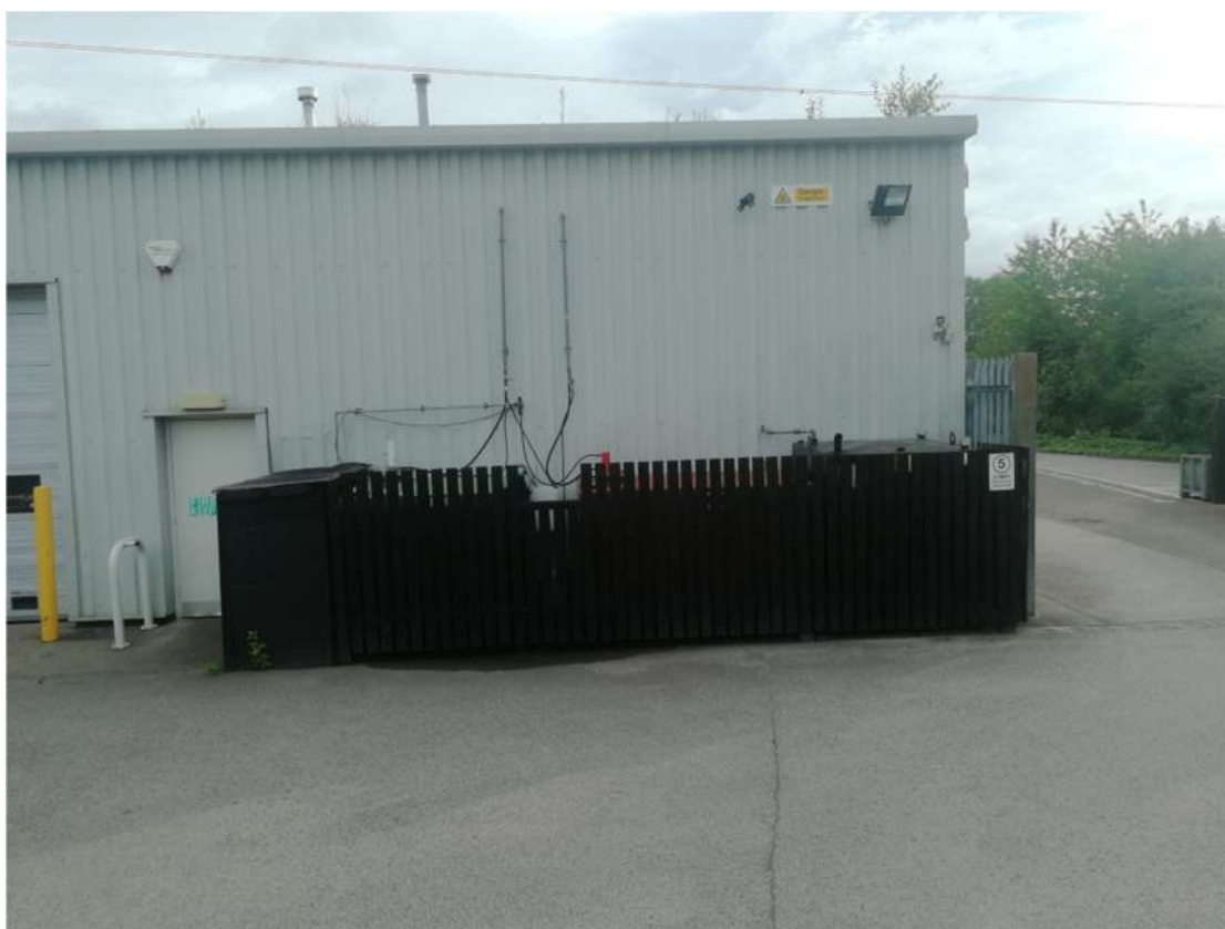
Photograph 10: Above ground oil storage tanks at southwest corner of main building.
