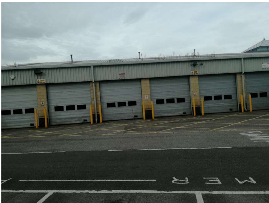
Photograph 6: Eastern face of the car showroom, facing west.
