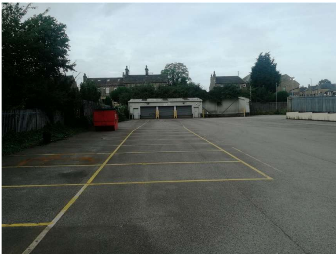
Photograph 16: Hardstanding across the western end of the site, facing west.
