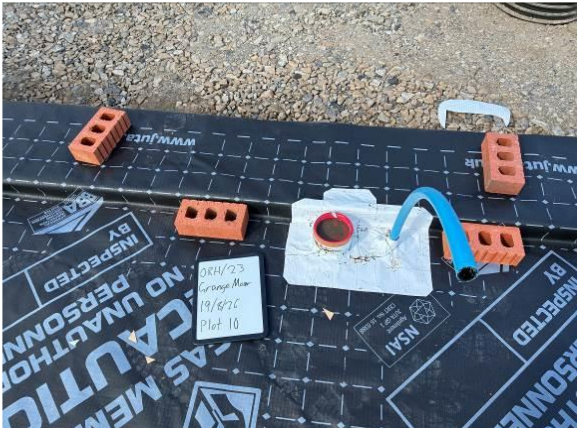
Photograph 6: Example of SAM being used to seal a double service entry on Plot 10. 19/8/26
