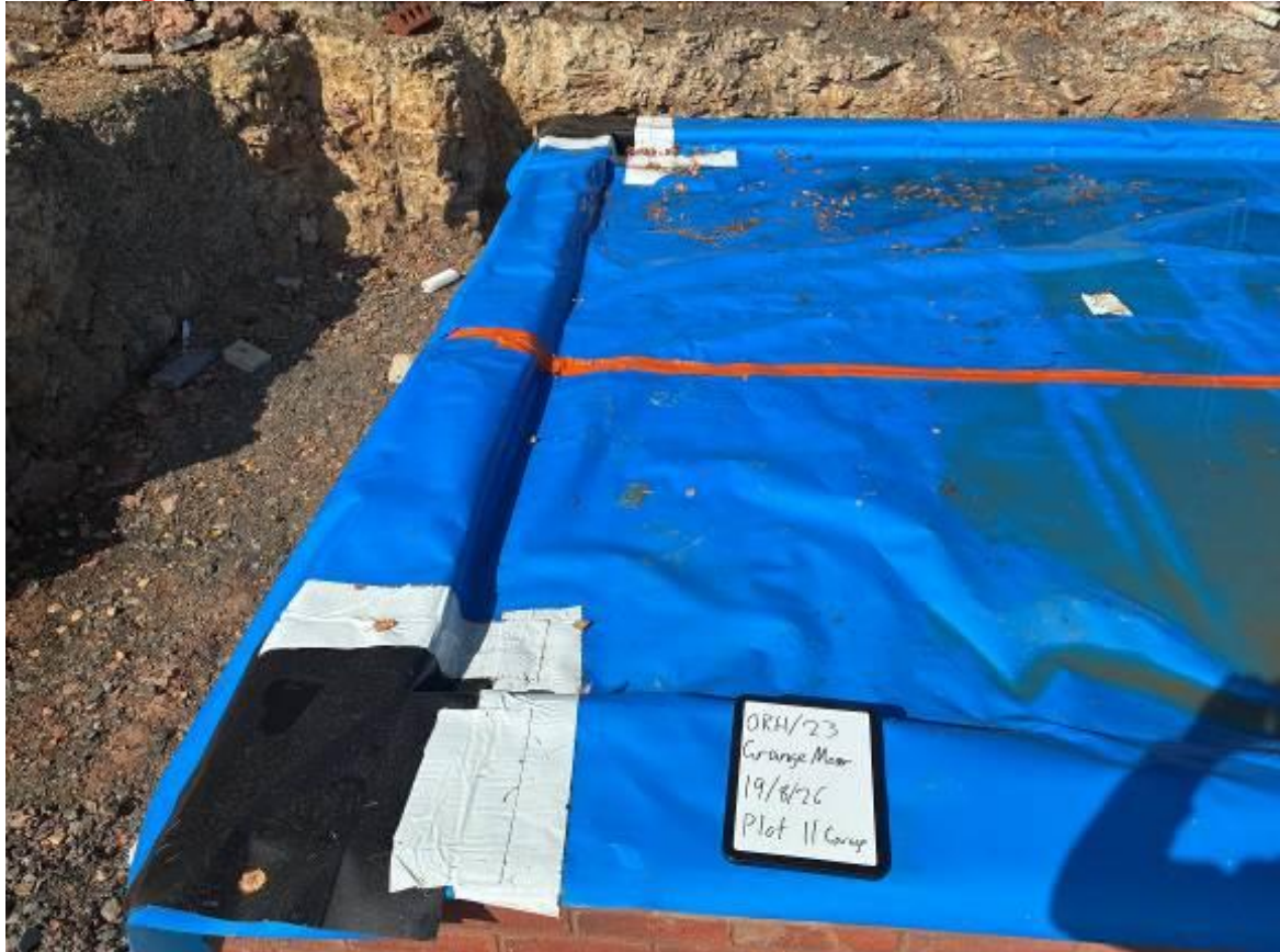
Photograph 3: Example of SAM detail being used on a corner of Plot 11 garage. 19/8/26
