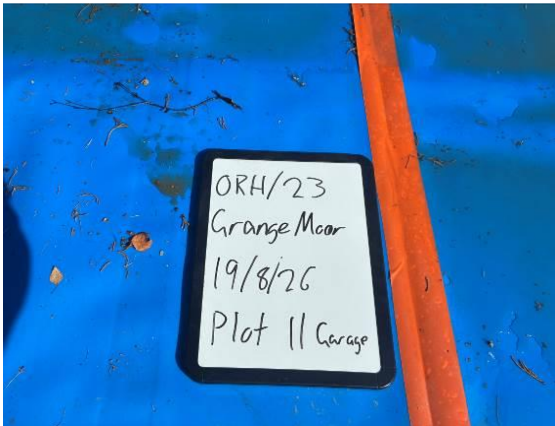
Photograph 4: View of double sided tape and lap tape connecting sheets of gas membrane together Plot 11 garage. 19/8/26
