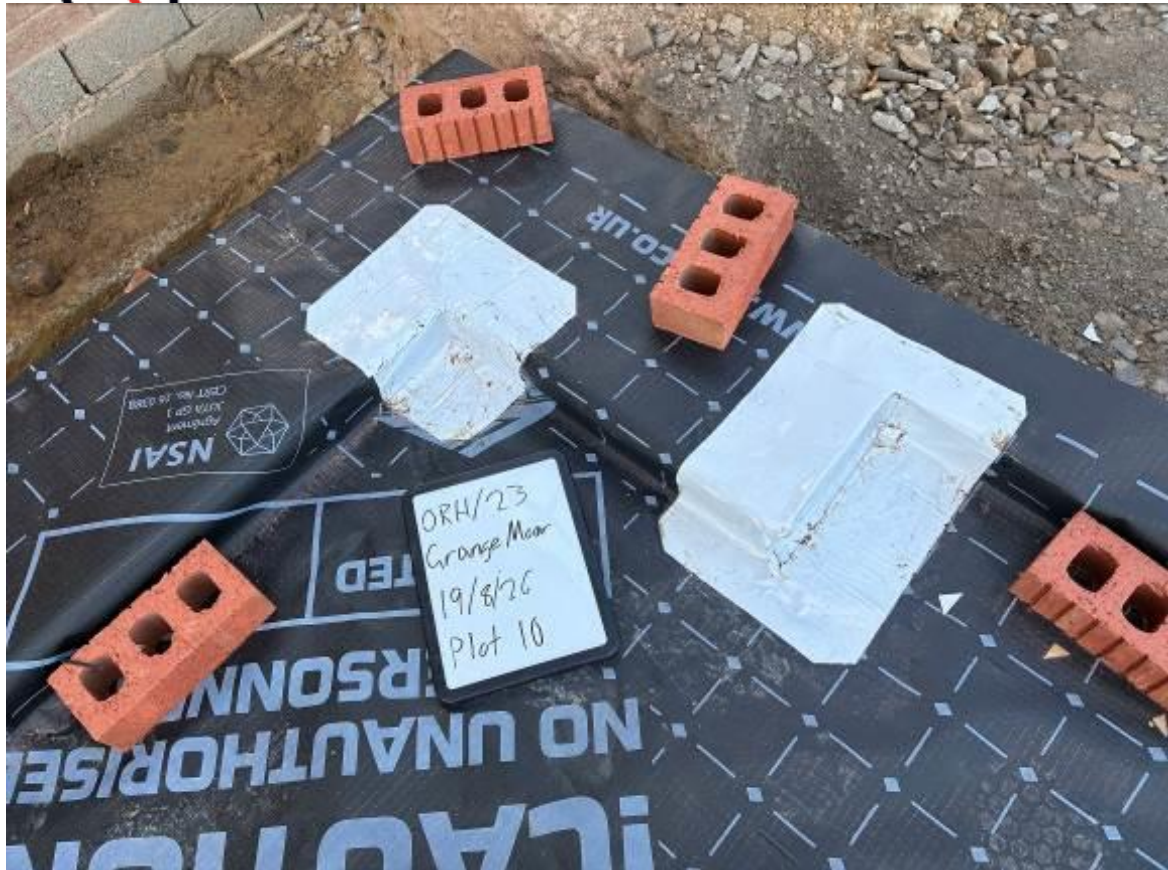
Photograph 7: Example of SAM detail being used on a corner of Plot 10. 19/8/26
