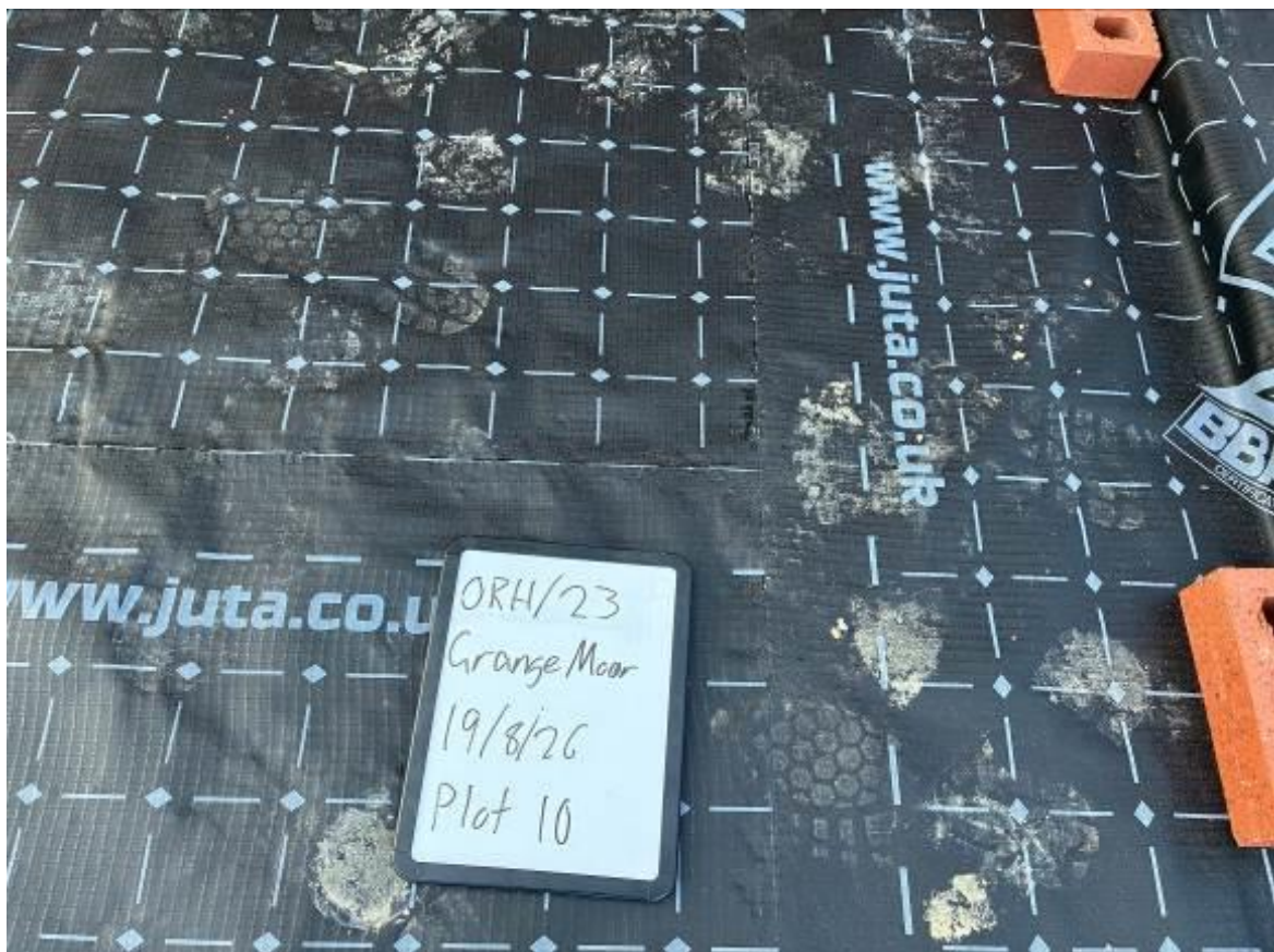
Photograph 8: View of heat welded joints connecting sheets of gas membrane together Plot 10. 19/8/26
