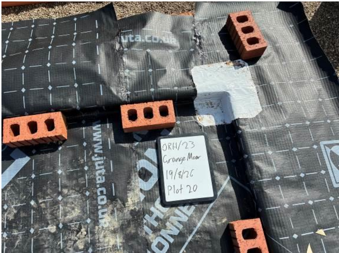
Photograph 10: Example of SAM detail being used on a corner detail of Plot 20. 19/8/26
