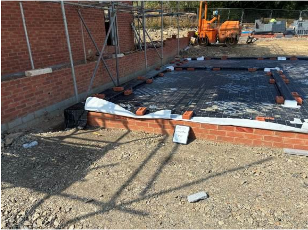
Photograph 13: View of evenly spaced periscopic vents on Plot 10. 19/8/26
