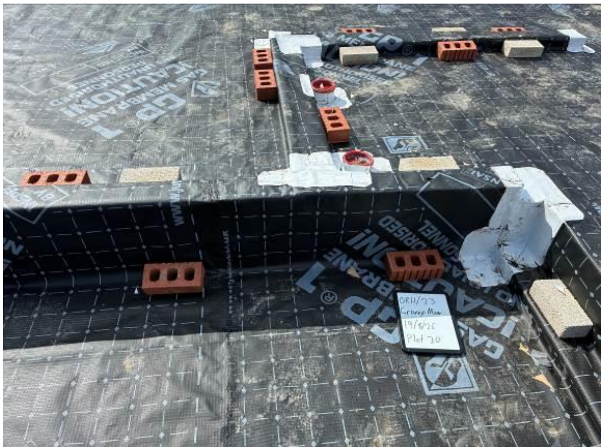
Photograph 12: View of heat welded joints connecting sheets of gas membrane together as well as the detail work of the transition to the garage which is a lower elevation on Plot 20. 19/8/26
