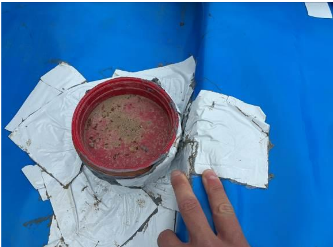
Photograph 2: Example of SAM being used to seal a service entry on Plot 11. 29/7/26
