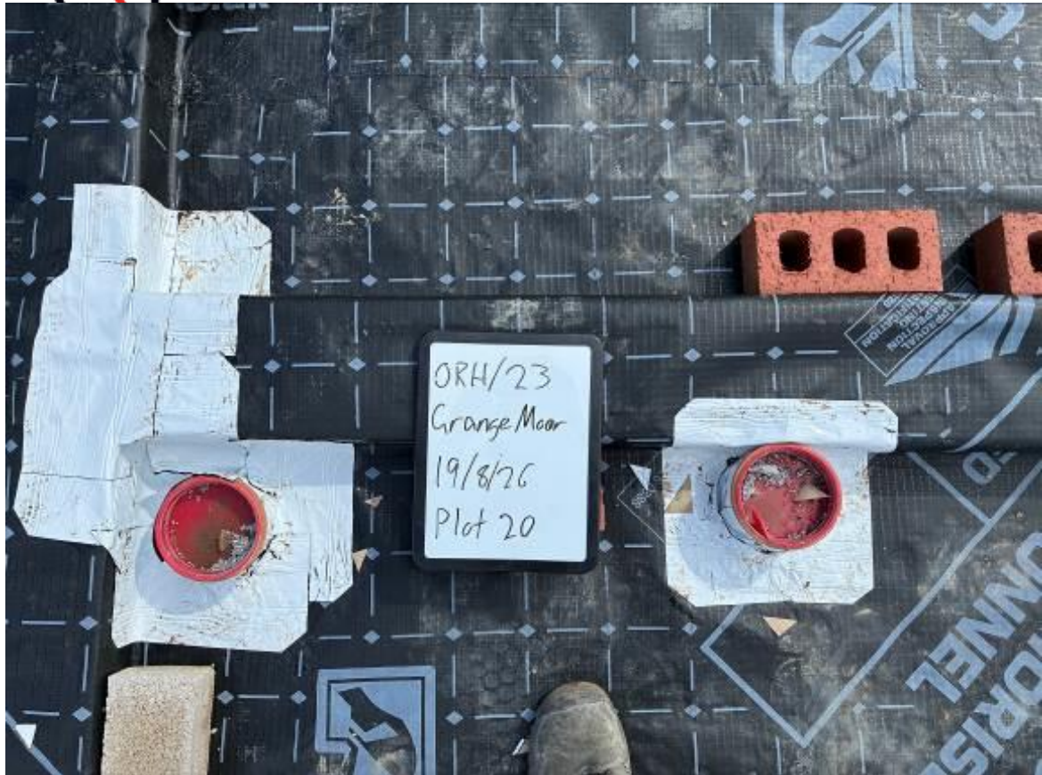
Photograph 11: Example of SAM being used to seal a service entry on Plot 20. 19/8/26
