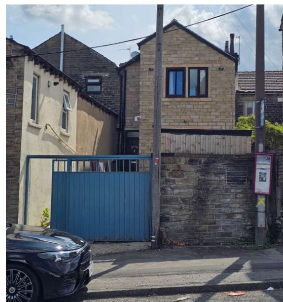
Front view of existing gate
