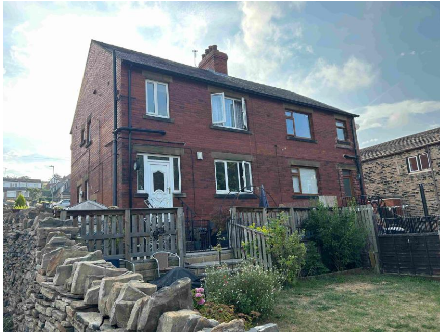
Photograph 2 – The rear of 41 and 43 Fenay Bridge Road. No.43 is the semi to the left hand side of the photograph.
