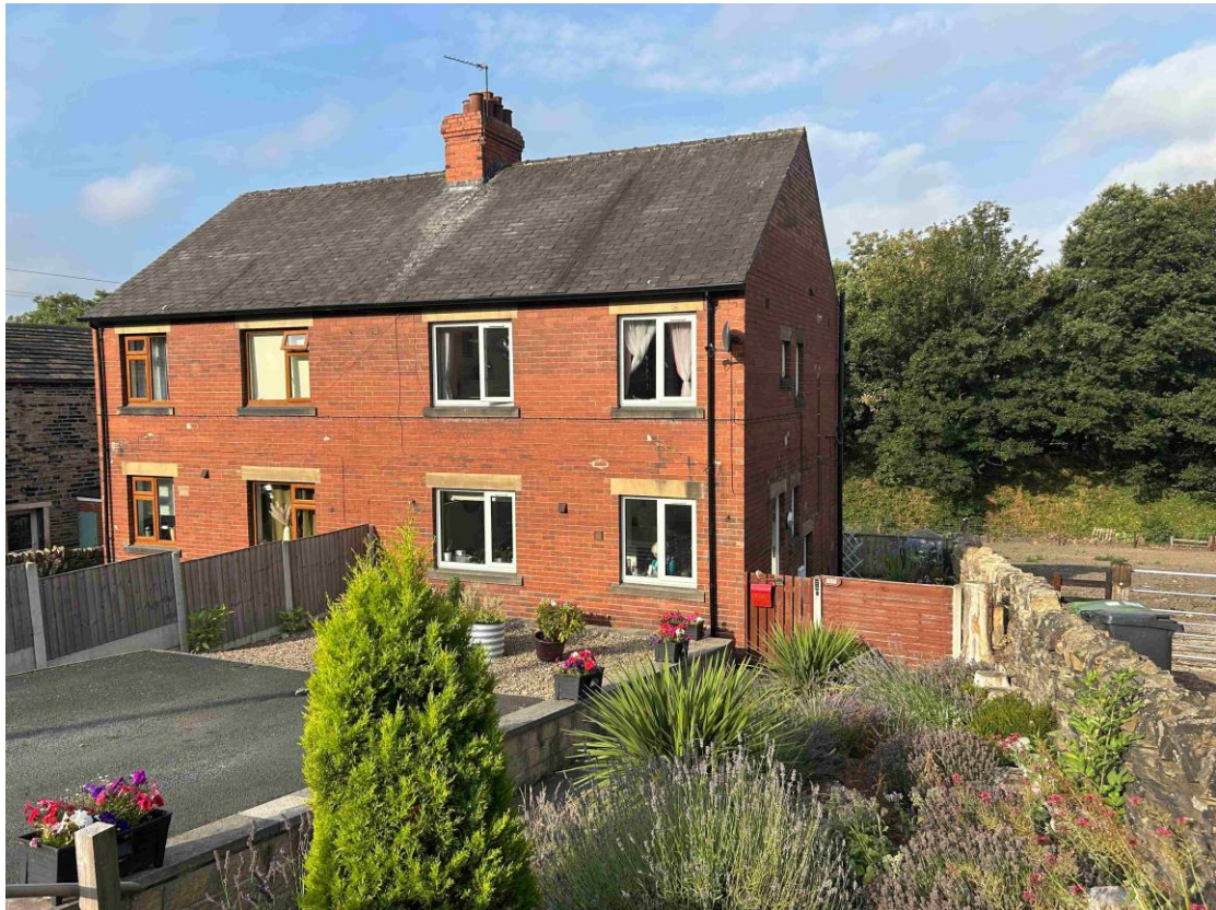
Photograph 1 - 41 and 43 Fenay Bridge Road. No.43 is the semi to the right hand side of the photograph.
