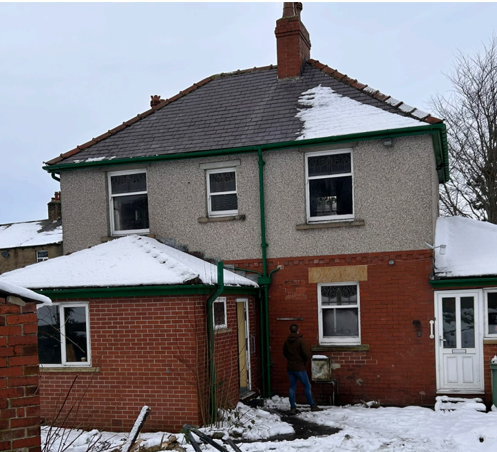
Photograph of existing blue slate roof of 5 Cumberworth Road.
