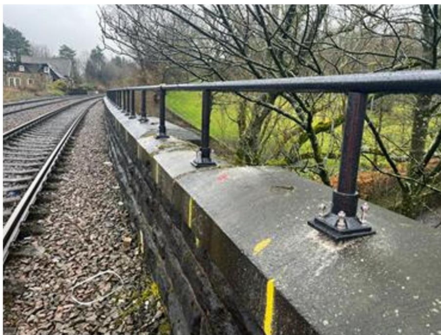
Insert 4-9 - Photo of comparable handrail installed at Uppermill (Saddleworth) Viaduct (MVL3/31) (Grade II Listed, NHLE 1068120)
