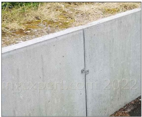
Flag on edge retaining wall under 400mm in height from ground level utilising paving to match plot paving
