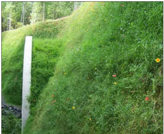
Gravitas Flex MSE geogrid reinforced, vegetated retaining wall for walls over 600mm
