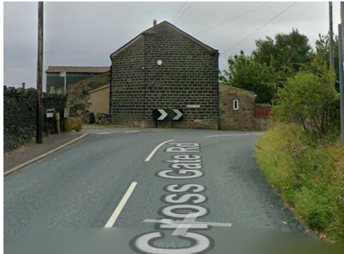
Approach From Cross Gate Road heading North-East.
