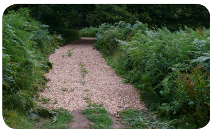
Step 1: Prepare Surface
