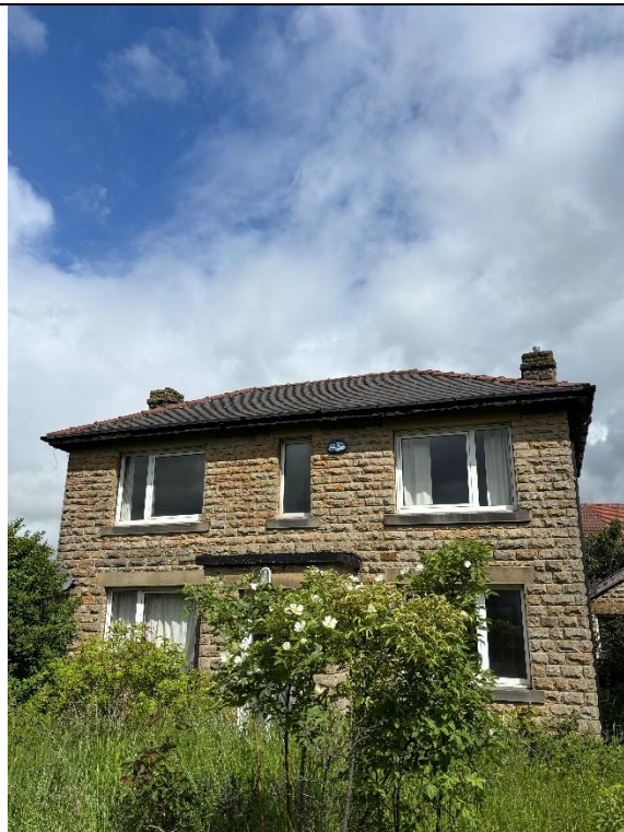
Photograph 12: View of the south facing elevation of the dwelling.
