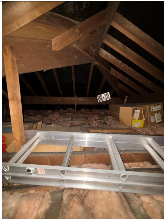
Photograph 16: View of the loft space. Timber beams and rafters support the roof felt lined loft space.
