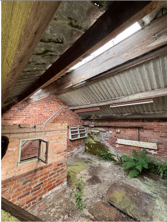
Photograph 9: Overview of the internal area of the garage.
