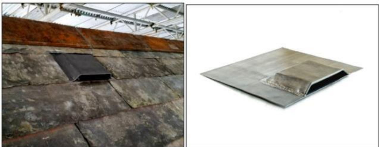
Figure 4.1: Image showing bat access slates
