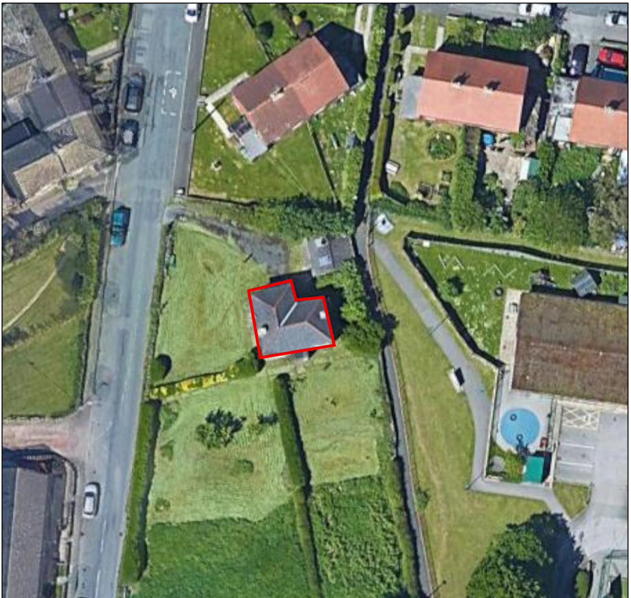
Figure 1.2: Aerial image of dwelling at Back Lane.
