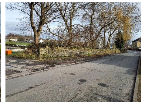
Figure 16 New Popplewell lane wall and road with curbs
