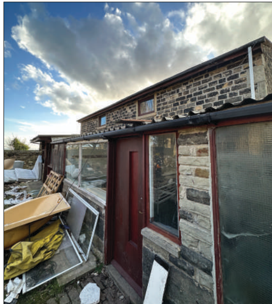
View towards the existing stone building.
