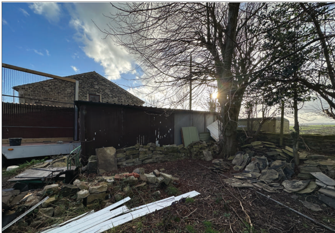
View of the existing stone building to be converted.
