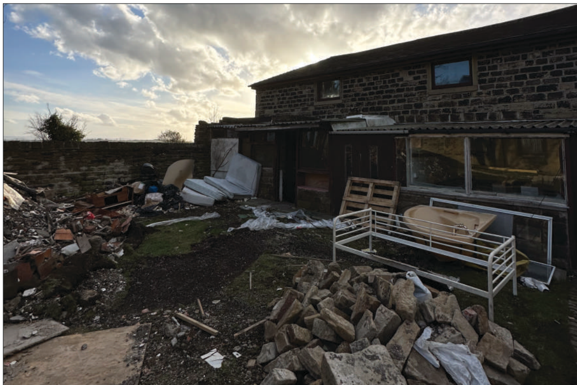
View of the existing stone building to be converted.
