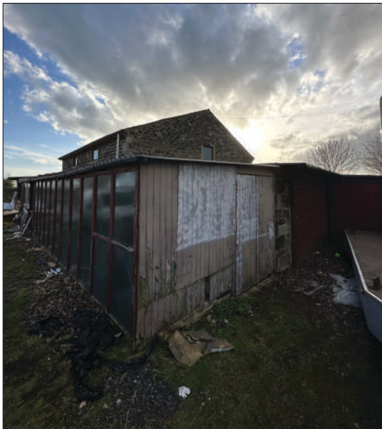
View towards the existing stone building.
