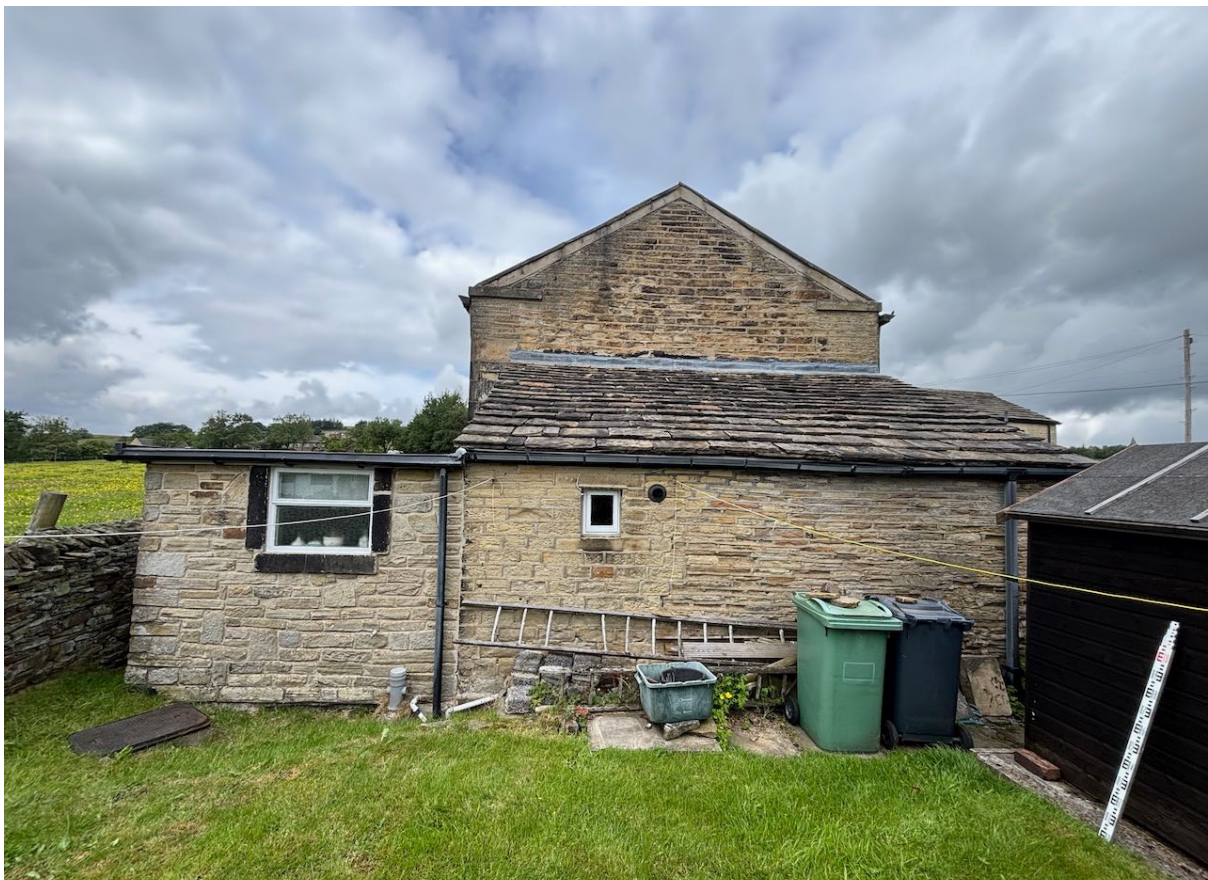
Figure 18: Photograph of the host dwelling showing the mismatched stone of the extensions
