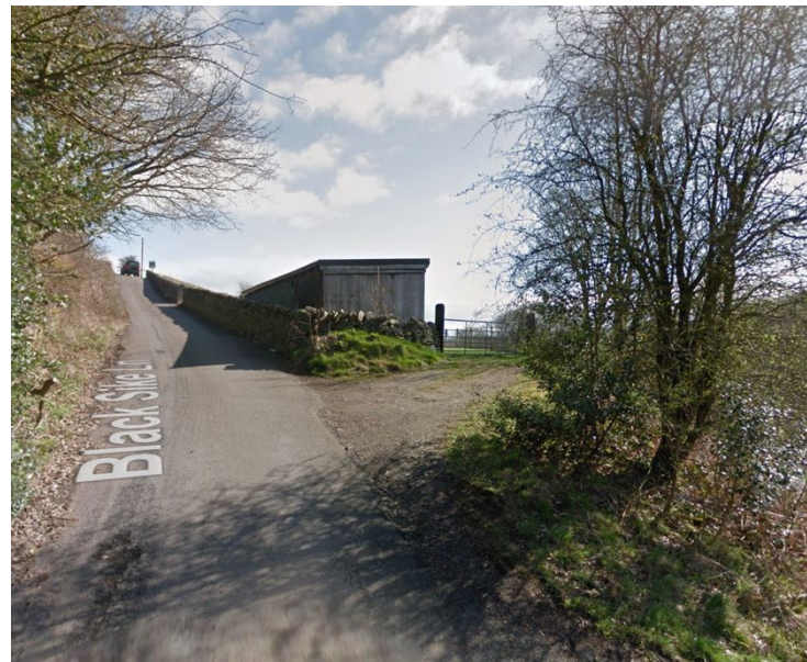
Figure 14: Barn on Black Sike Lane
