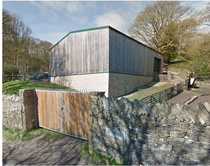
Figure 12: Barn on Black Sike Lane
