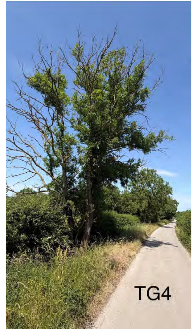
TG4 - above - a row of ash in decline from ADB over a road, which is also a farm access track and PROW.
