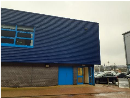
Figure 6 view of building from south
