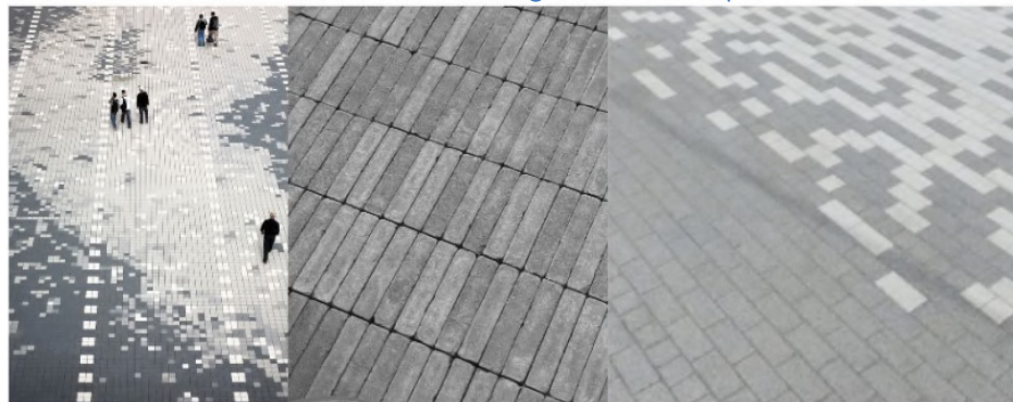
Paving transition at pedestrian entrances
