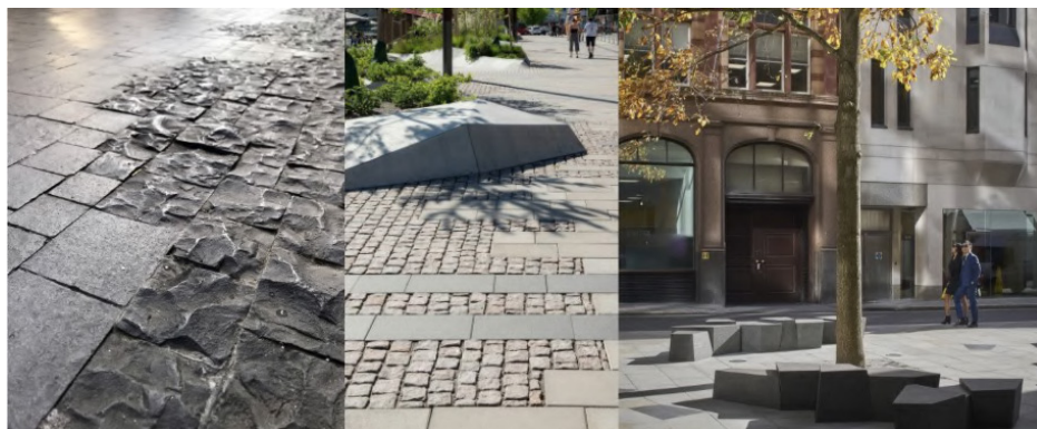
Deterrent paving and raised edges underneath the low overhangs
