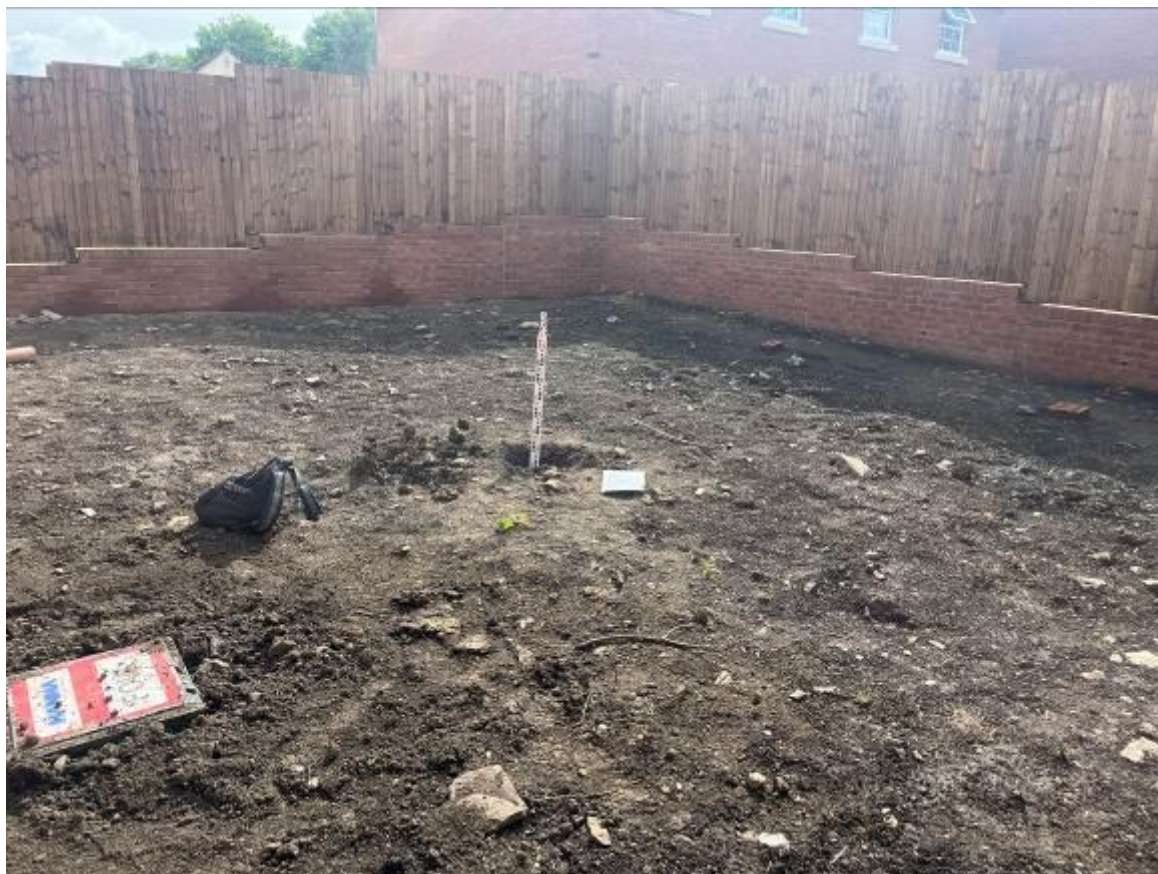
Photograph 1: General view of the pit dug in the rear garden of Plot 20.
