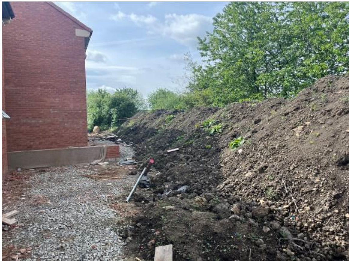
Photograph 4: View of the topsoil stockpile stored in the rear gardens of Plots 15 to 19
