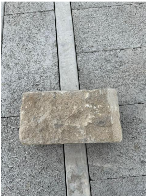
Drafted corners for all reveals and corners
