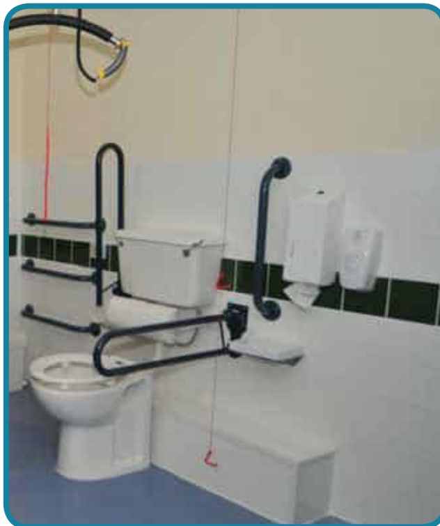
Drop-down rails on both sides of the WC can be folded up when not needed or dropped-down into horizontal position for support. The black grabrails contrast visually against the pale background
