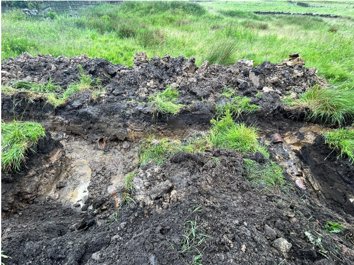
Figure 3 Two existing clay pipes
